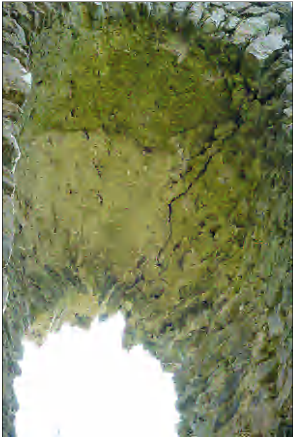
Figure 2.55. Window 1.2, plaster in underside of window embrasure, from SW (F. Coyne).
