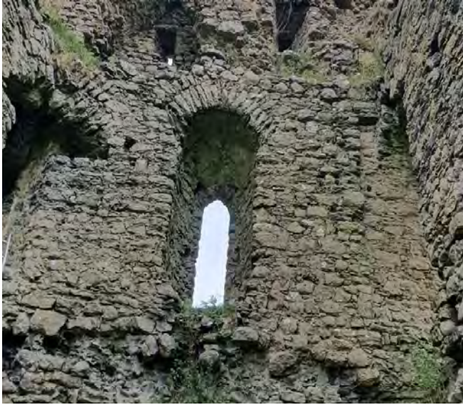
North eastern elevation showing stairs ope and squinch on the left.
