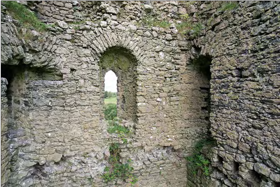
Figure 2.59. Window 1.4, plaster in underside of window embrasure, from SW (F. Coyne).
