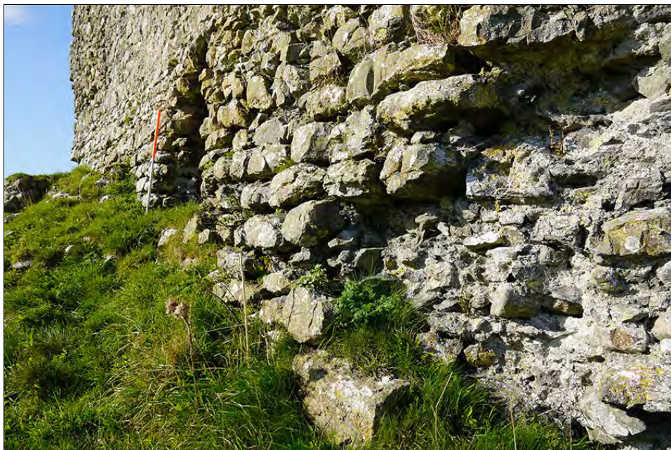
Figure 2.40. Robbed out base batter on NE wall. Note intact batter to rear (F. Coyne).
