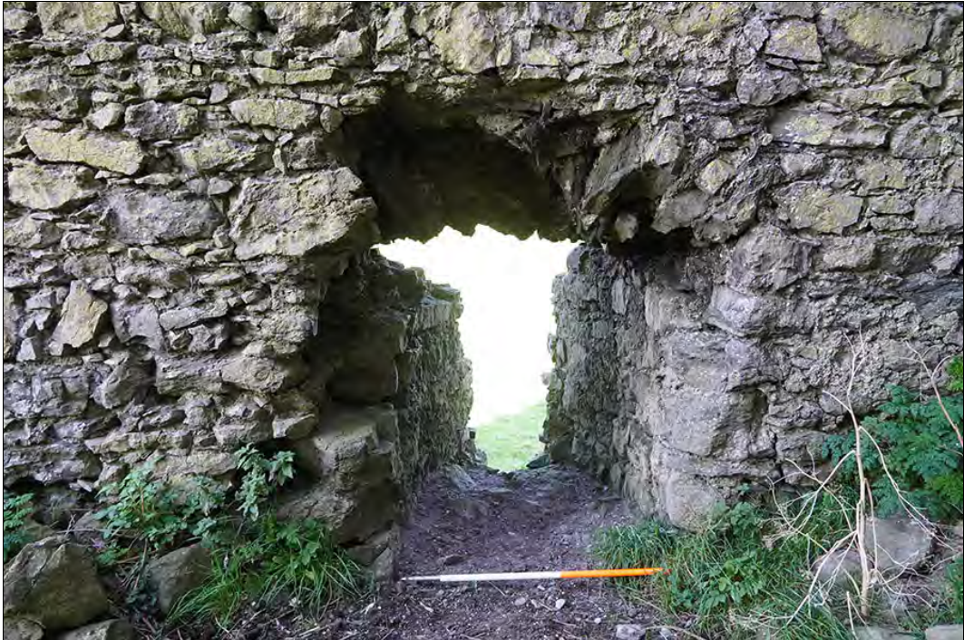
Figure 2.48. Window 5, note slot for timber lintel and robbed out flat arch, from NW (F. Coyne).
