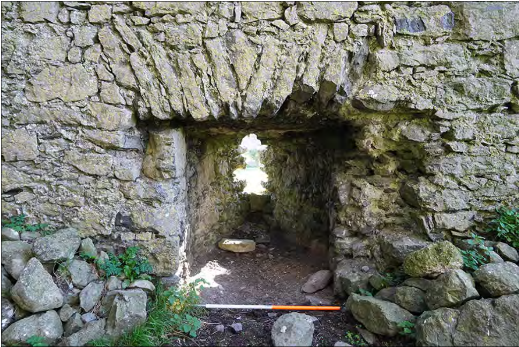
Figure 2.44. Window 2, note slot for timber lintel, from NW (F. Coyne).
