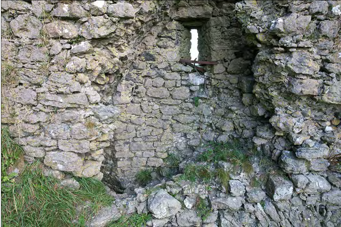
Figure 2.64. Loop 2.1 in stairwell on 2 nd floor, from SW (F. Coyne).
