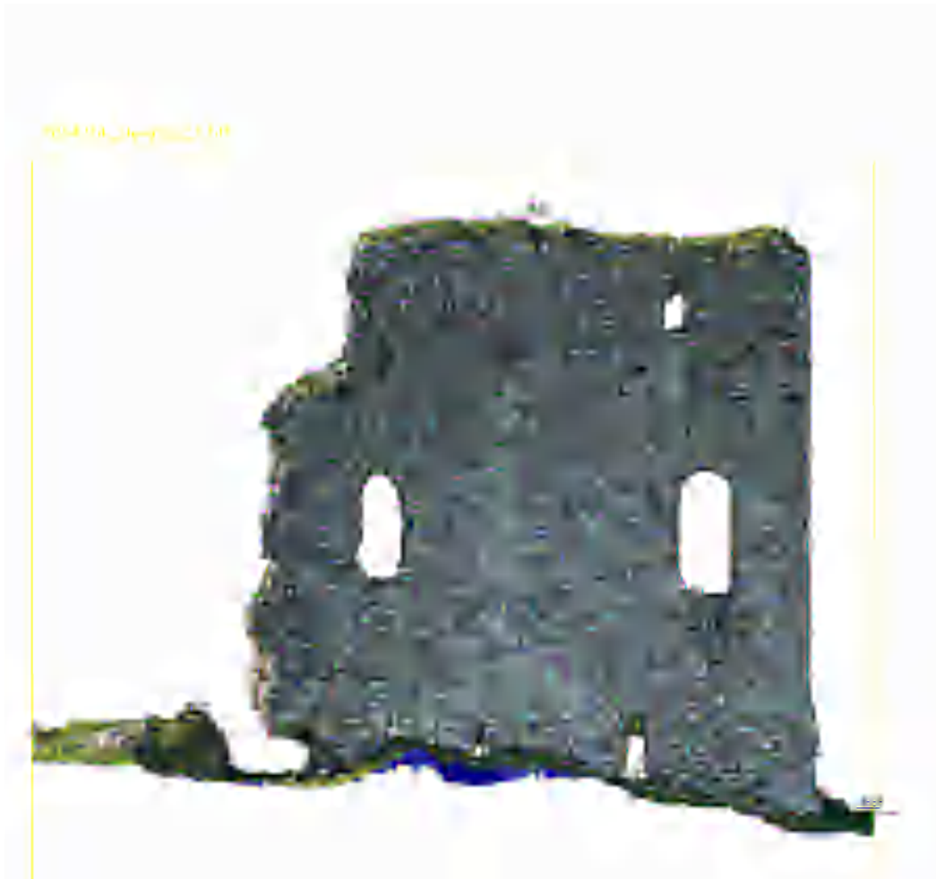
View of South-east elevation with first floor entrance on the right
