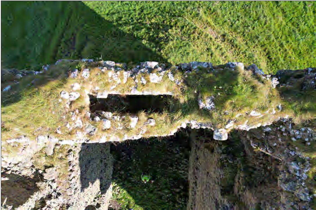
Figure 2.63. Access from stairs to parapet, view from above (F. Coyne).
