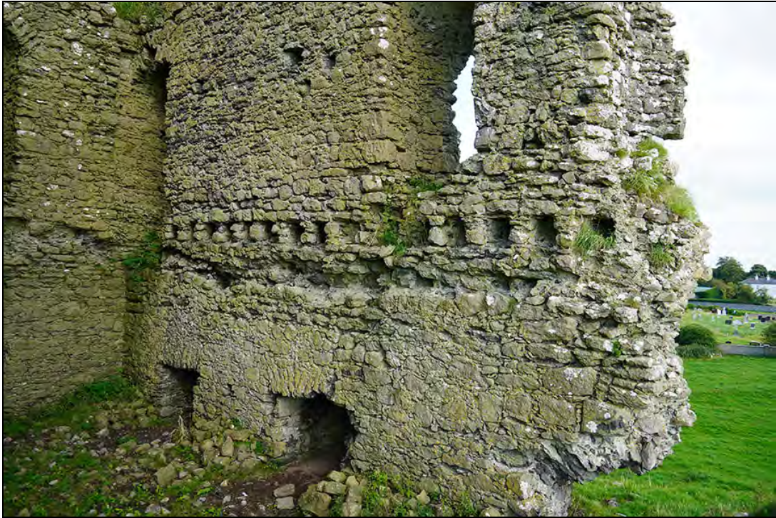
Figure 2.35. Scar in masonry and beam sockets, from W (F. Coyne).
