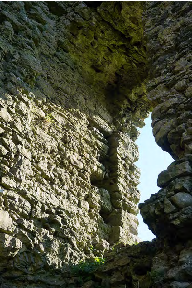
Figure 2.57. Door ope 1.3, from W. Note drawbar socket. (F. Coyne).
