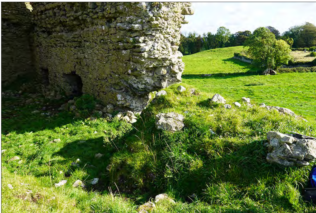
Figure 2.72. fallen masonry, from W (F. Coyne).
