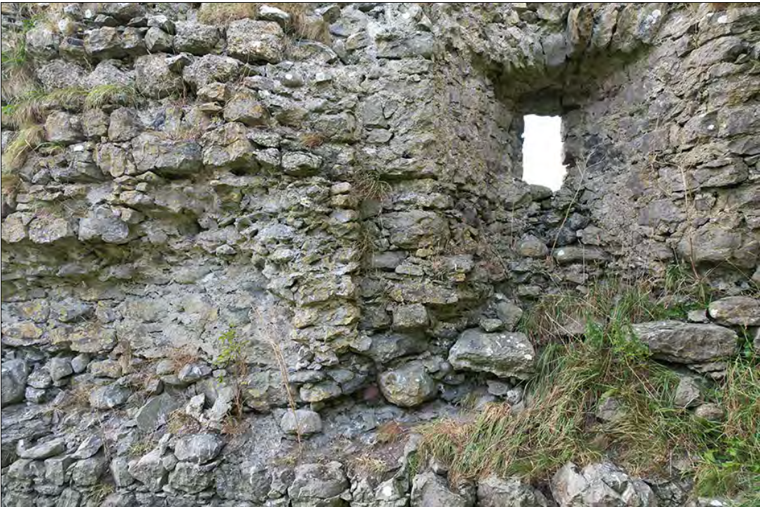
Figure 2.67. Window 2.4, from SW (F. Coyne).
