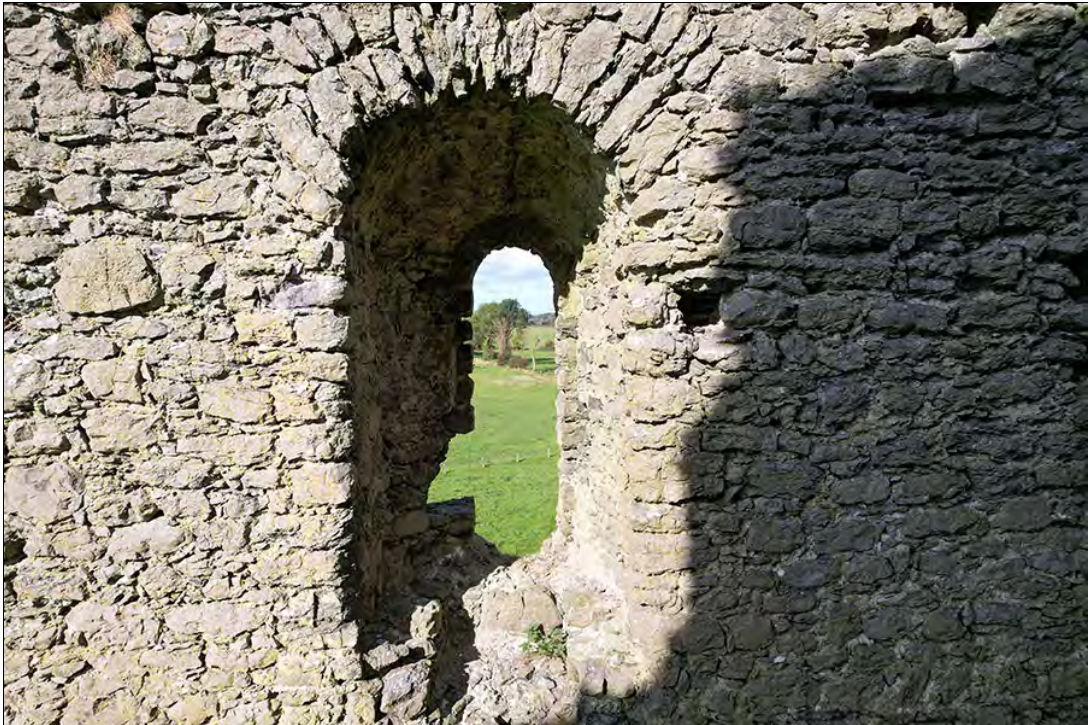
Figure 2.61. Window 1.6, plaster in underside of window embrasure, from SE (F. Coyne).
