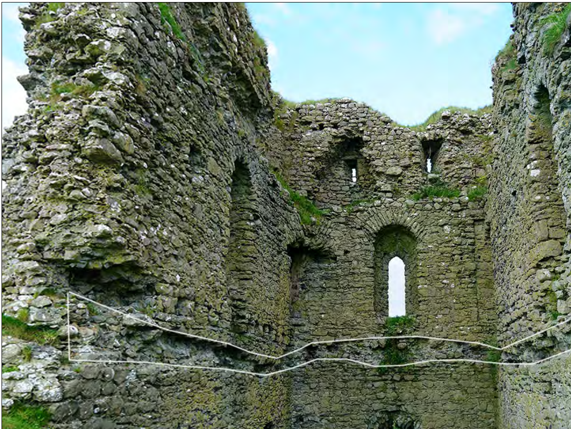
Figure 2.34. Scar for possible vault indicated, from SW (F. Coyne).
