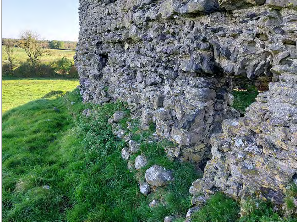
Figure 2.39. Robbed out base batter on NW wall (F. Coyne).
