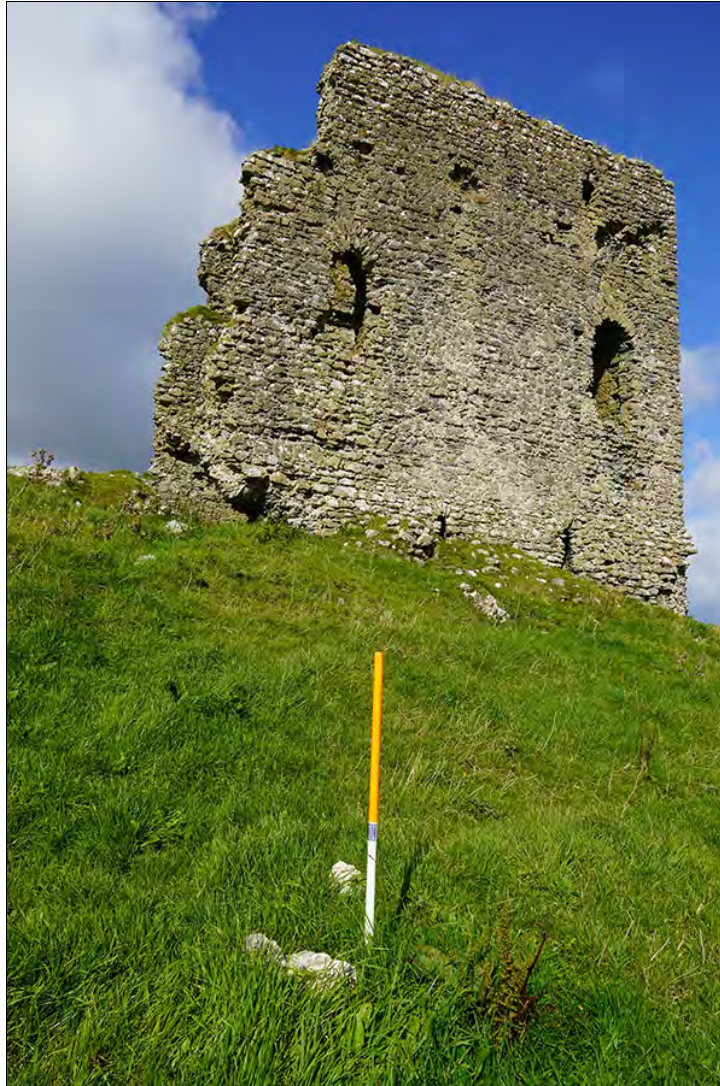
Figure 2.73. Castle with fallen masonry in immediate foreground, from S (F. Coyne).
