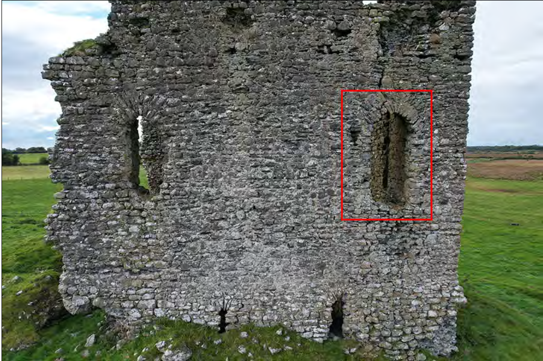
Figure 2.58. External view of door ope 1.3, from SE (F. Coyne).
