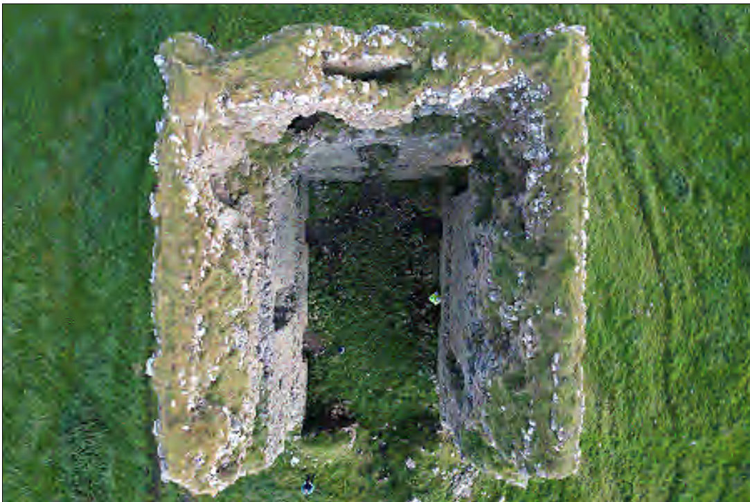
Figure 2.29. Vertical view of Moylough Castle (F. Coyne).
