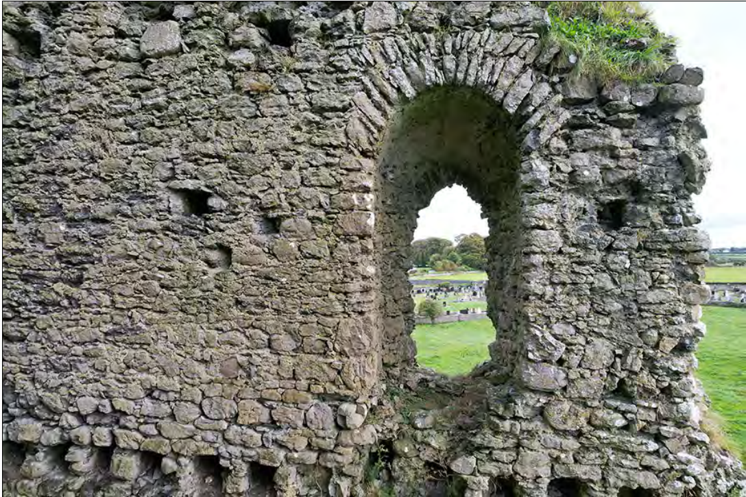
Figure 2.54. Window 1.2, from SW (F. Coyne).
