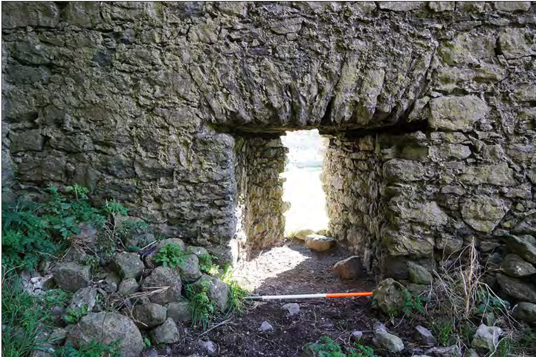
Figure 2.46. Window 3, note slot for timber lintel, from NW (F. Coyne).
