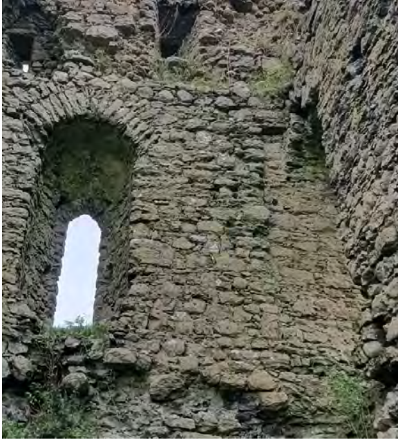
Interior view showing entrance door recess on the right
