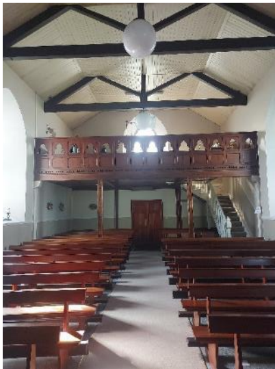
Photograph 43: Gallery and roof in Glinsk Church
