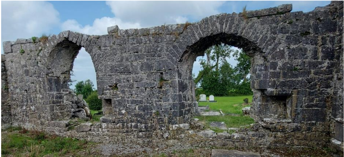
Photograph 32: Two window openings and associated aumbry in the east wall of the side chapel at Ballinakill
