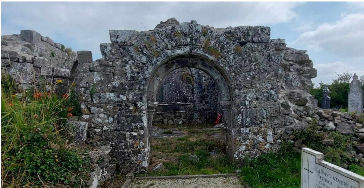
Photograph 31: Entrance doorway to side-chapel at Ballinakill
