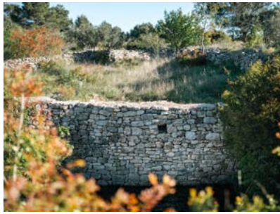
Restoration of a dry stone pond, Zlarin, Croatia.
