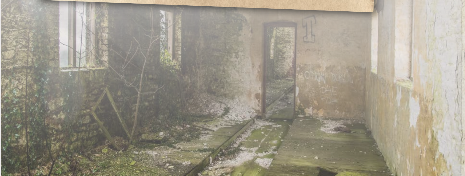
A sleeping area in a ruined workhouse; note the platforms on either side of the aisle where the straw mats used to be. Source: Adobe Stock
