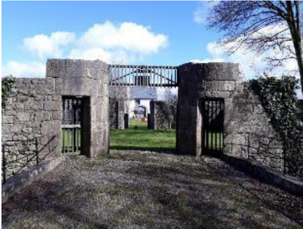
Photograph 92: Bridge at Brooklodge
