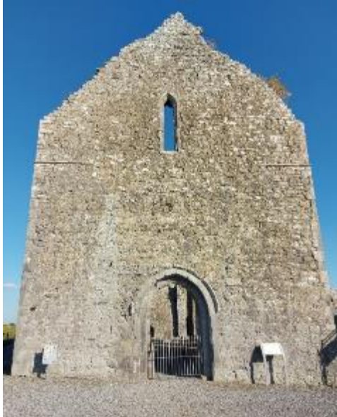
Photograph 8: The west gable and doorway
