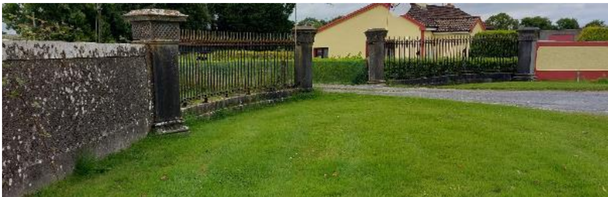
Photographs 84- 86: Moyne House Gateway
