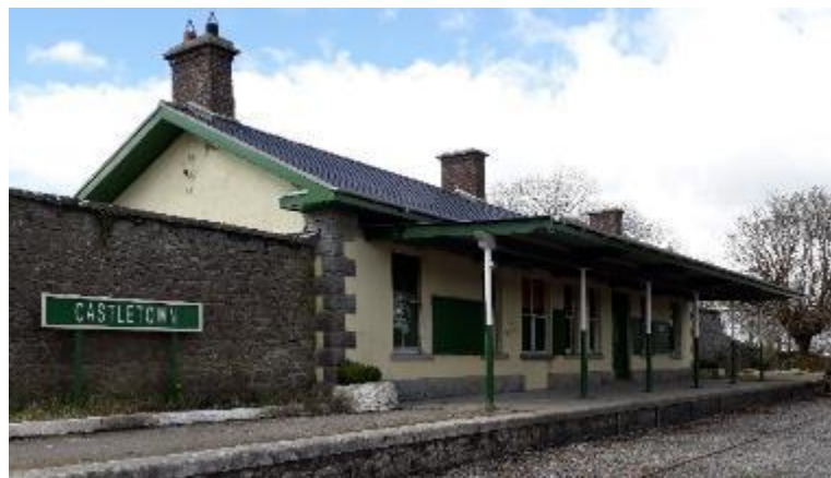
Photograph 123: Ballyglunin Station rear elevation.
