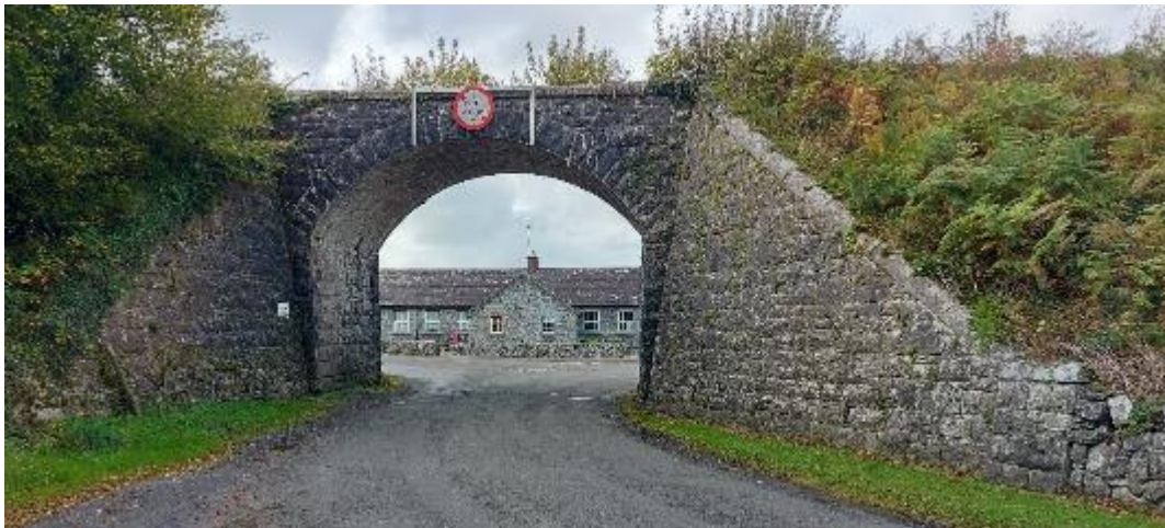
Photograph 121: View through Crumlin Bridge to former Crumlin National School
