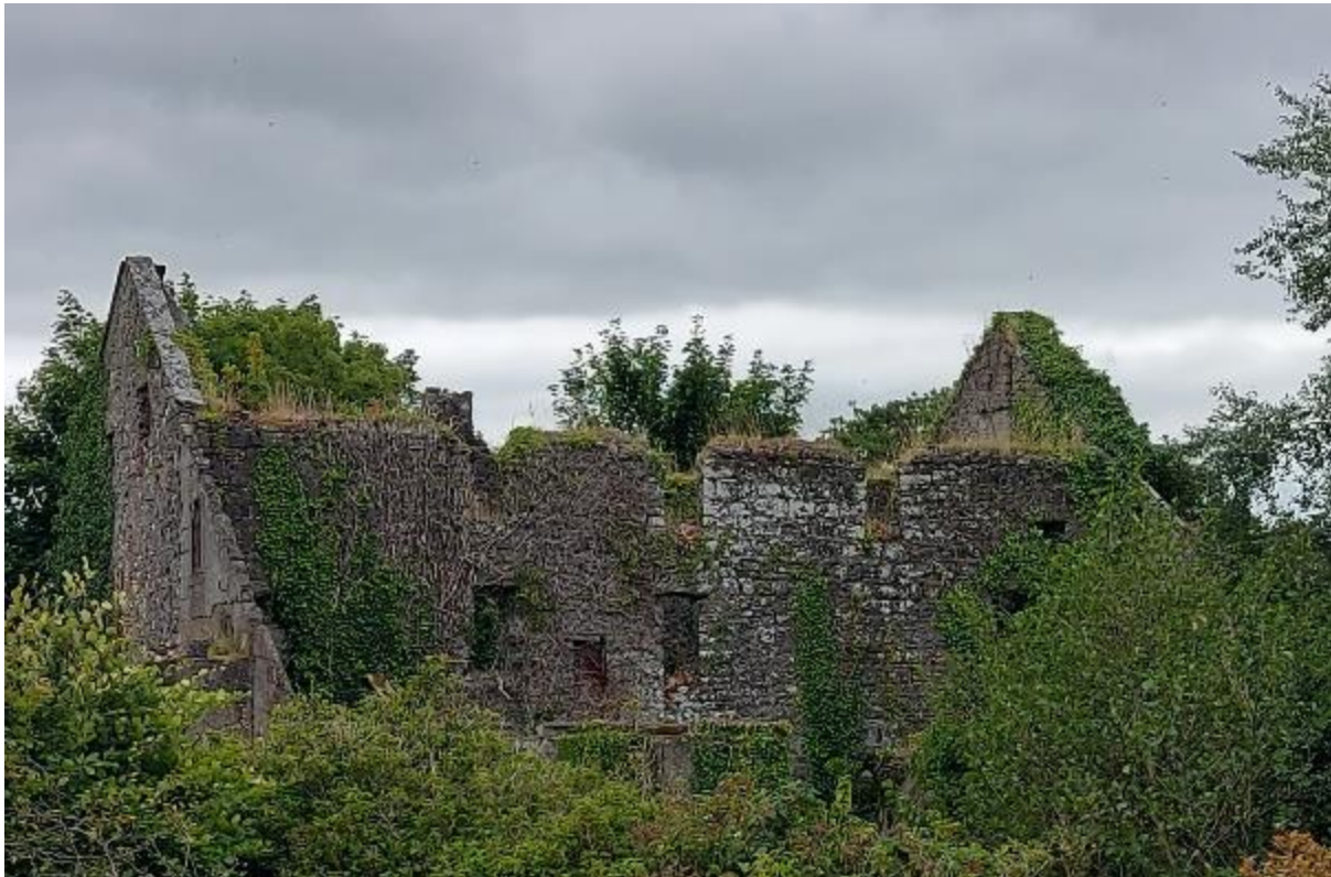
Photograph 104: View of Abbey Mill today
