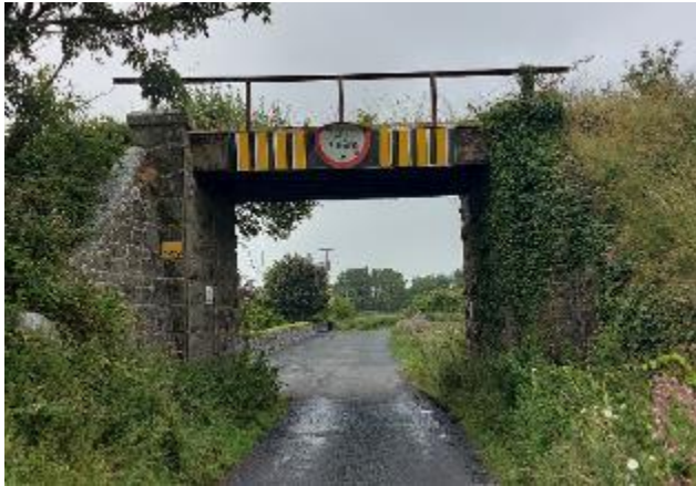
Photograph 119: Doonbeg Railway Bridge
