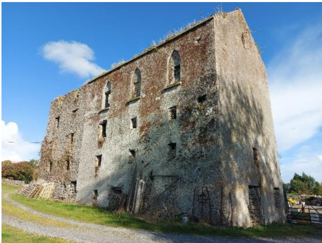
Photograph 98: Moyne Mill today viewed from the south.
