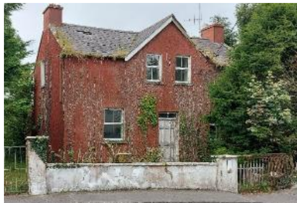
Photograph 114: Barnaderg School Teachers Residence
