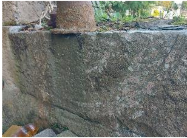
Photograph 102: Incised mark of former mill wheel on wheel pit wall
