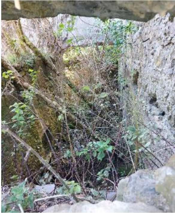
Photograph 101: View into the wheel pit from the mill race arch
