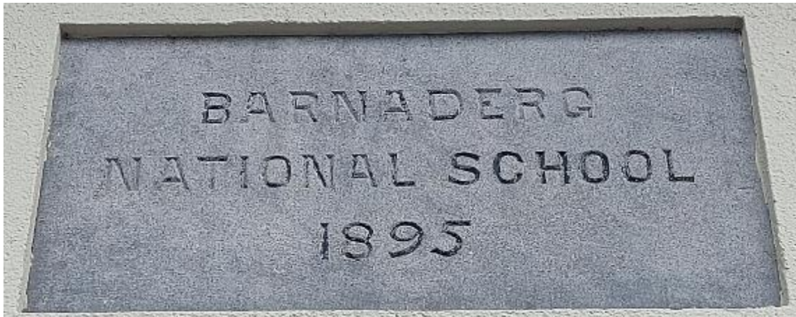
Photograph 110: Datestone for Barnaderg National School which today functions as the Community Centre
