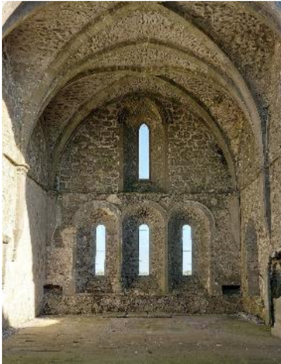
Photograph 13: The Chancel with ribbed vaulted roof and east window
