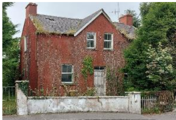
Photograph 115: Barnaderg School Teachers Residence
