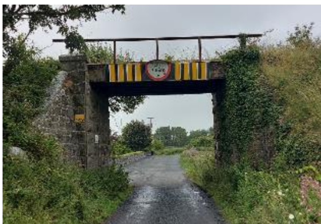
Photograph 120: Doonbeg Railway Bridge
