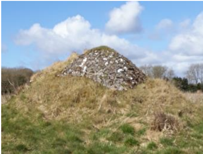
Photograph 93: View of rear of Ice House
