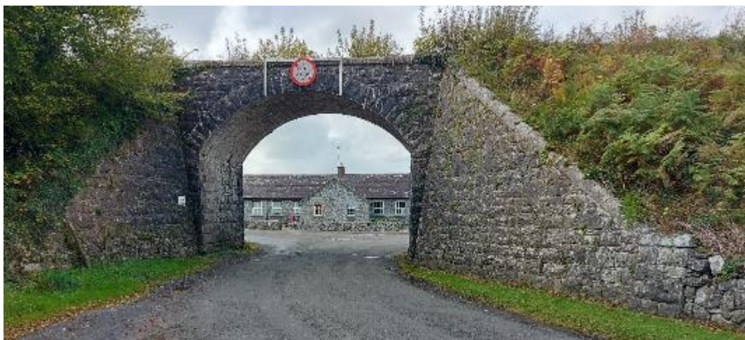
Photograph 122: View through Crumlin Bridge to former Crumlin National School
