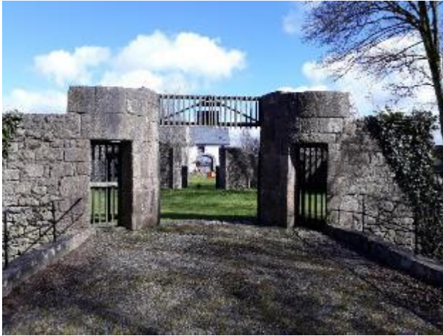
Photograph 92: Bridge at Brooklodge
