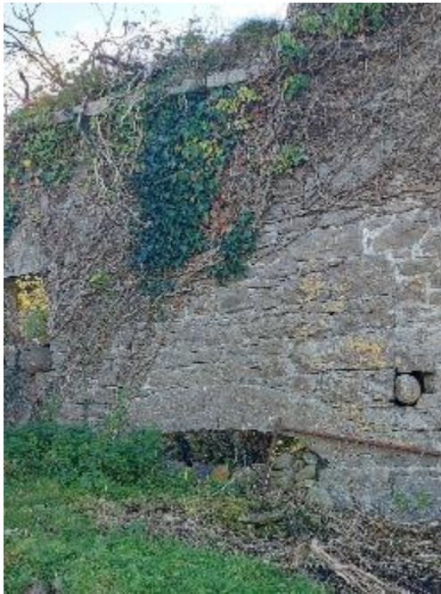
Photograph 99: arch where water entered the wheel pit Photograph 100: Section of former mill race wall
