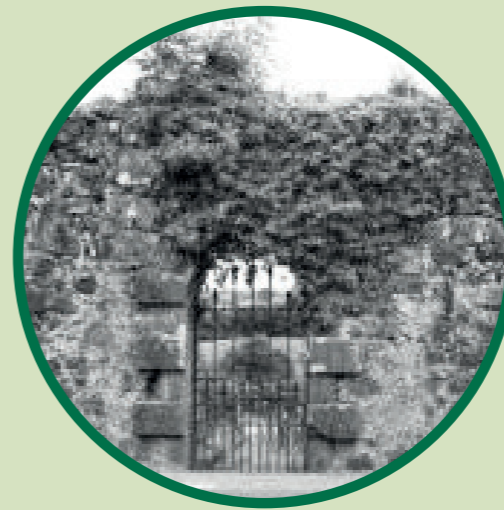
▲ Danesfield House garden walls and gate, 2016
