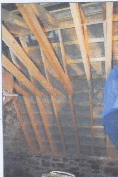
Plate 15 Parging, during application.
