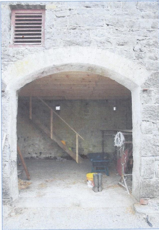
Plate 4 Stairs and ceiling joists, viewed from front of barn.
