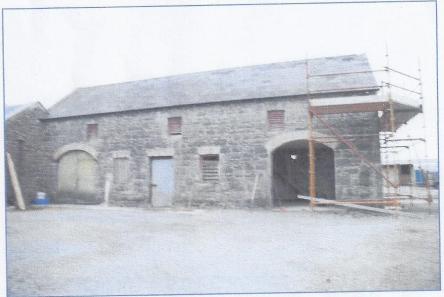
Plate 10 Re-slating complete, from front.
