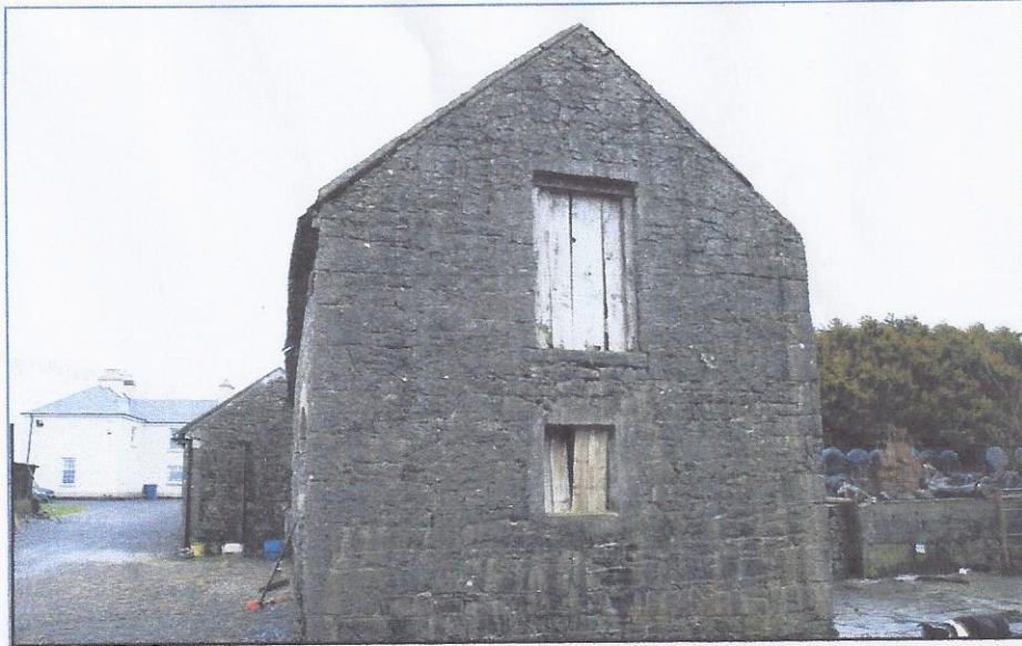
Plate 3 West gable of stable building, prior to works commencing.
