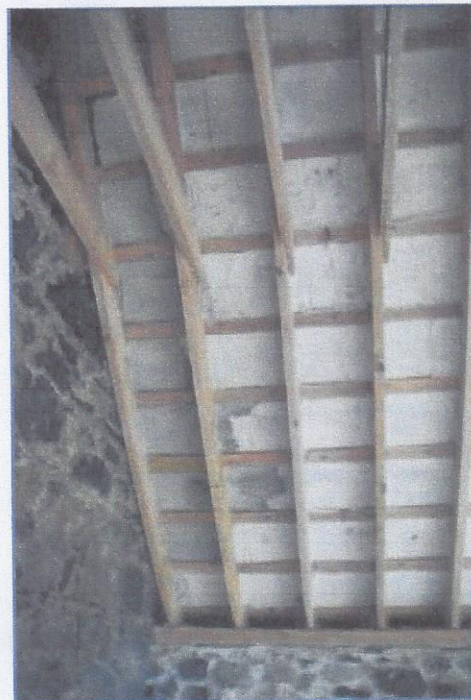
Plate 18 Interior of small barn, showing patching to parging, following completion.
