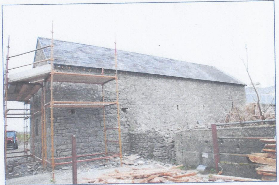
Plate 11 Re-slating complete, from rear.
