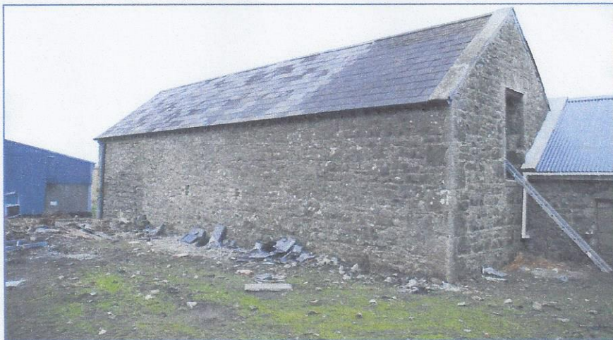
Plate 22 Rear of building, following completion of works.
