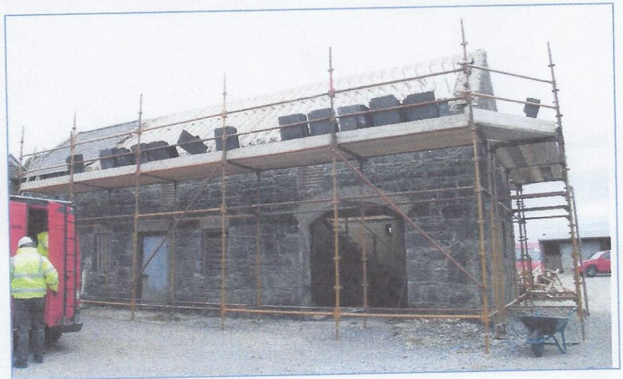
Plate 9 New rafters to building, from front.
