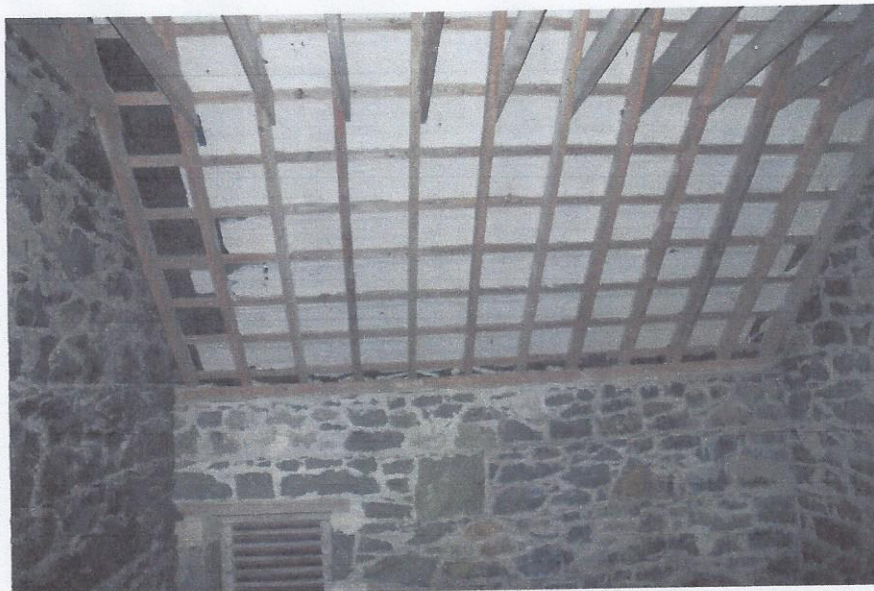
Plate 13 Interior, small barn, showing no alteration.
