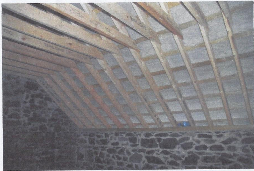
Plate 16 Parging, rear pitch, main barn, following completion.
