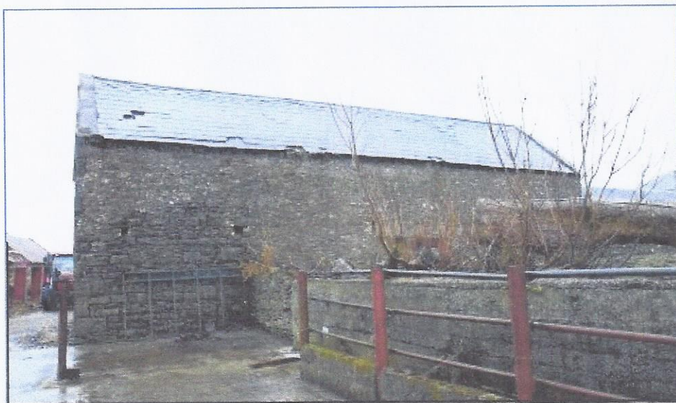
Plate 2 Stable building, from south, prior to works commencing.
