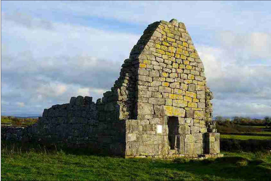
Figure 2.13. Early church at Killeely built in cyclopean masonry style
