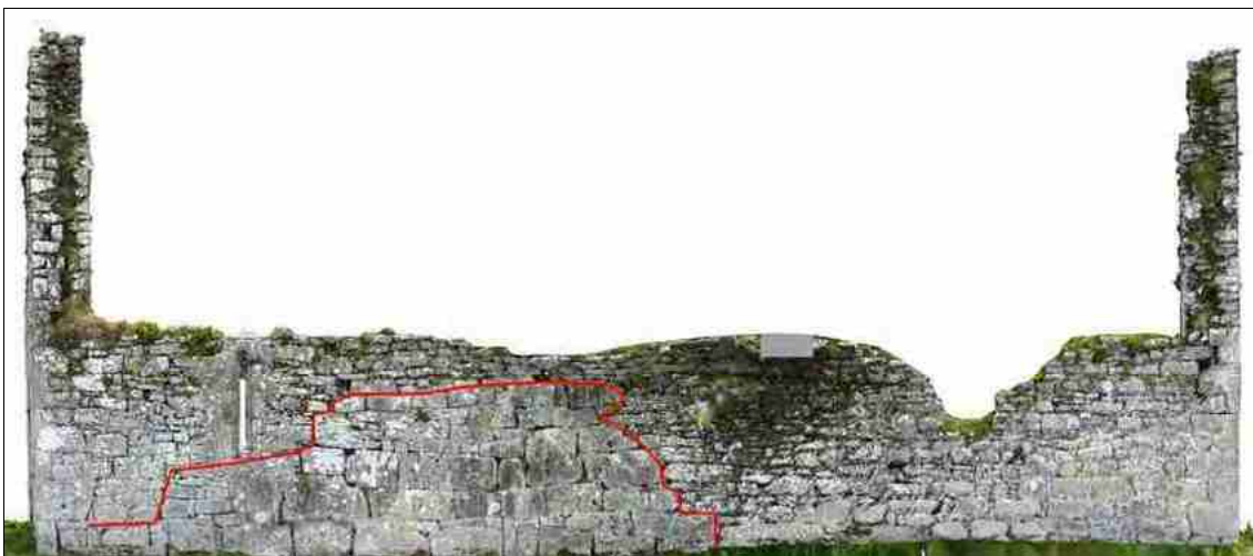
Figure 2.16. Elevation of exterior N of church wall showing cyplopean masonry(after OSECM, annotated by writer)
