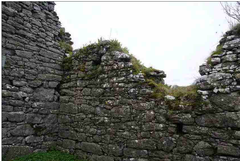
Figure 2.51. Joist holes in N wall, possible indication of a priest's residence, from S..
