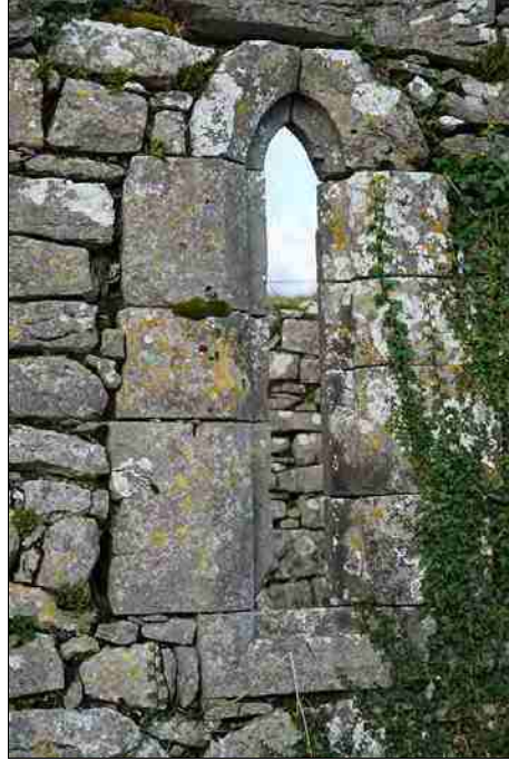
Figure 2.36. External view of window in S wall, from S.
