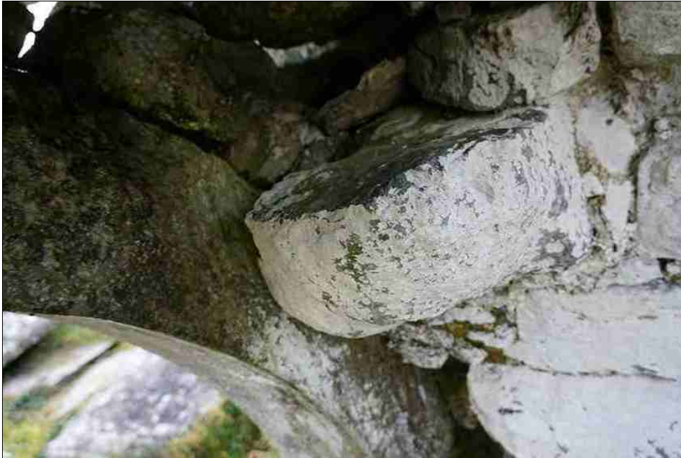
Figure 2.18. Detail of hanging eye, from NW.
