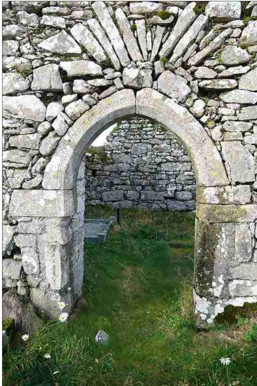
Figure 2.42. Church door, from S.
