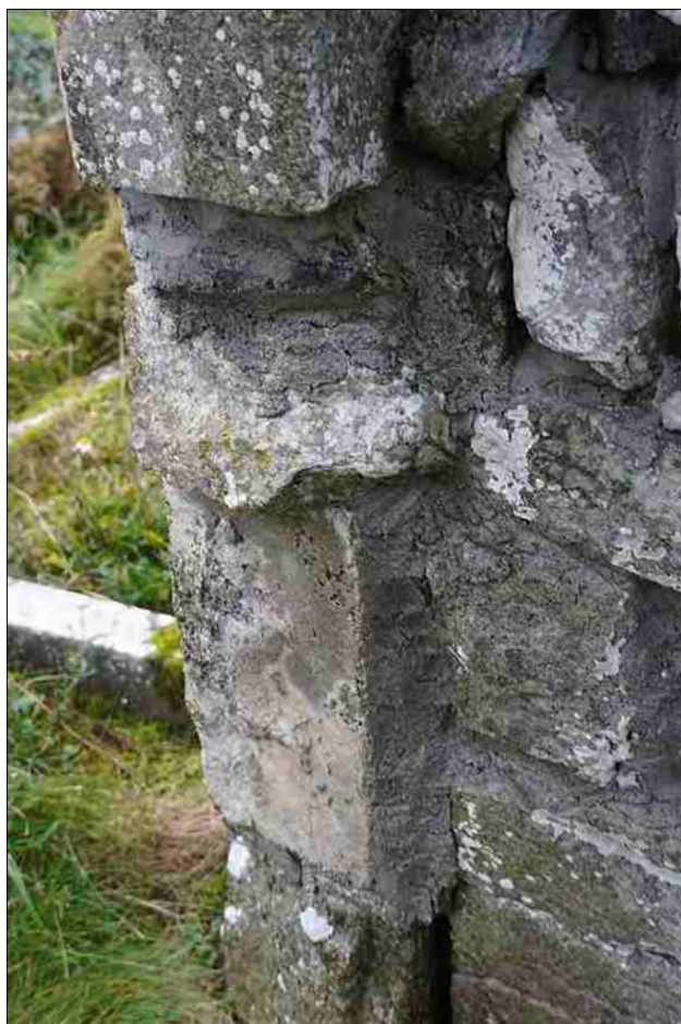
Figure 2.46. Concrete repairs on W side of door. Original door jamb missing at this side.
