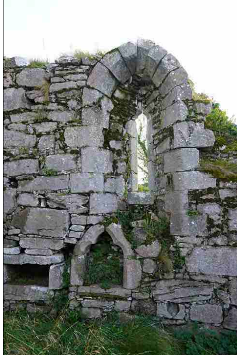
Figure 2.37. Internal view of window in S wall, from S. Note aumbrey and piscina below.
