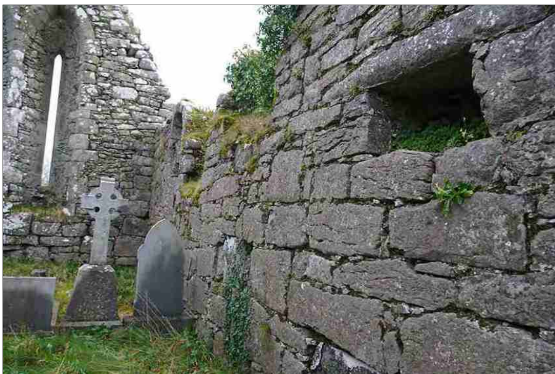
Figure 2.41. Wall niche/cupboard, from W.
