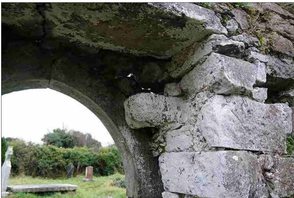
Figure 2.45. Hanging eye for door on W side of entrance.
