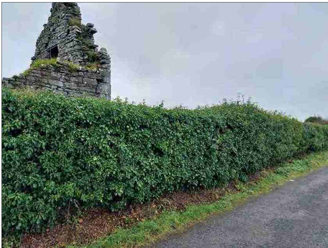
Figure 2.55. Graveyard wall, from NE.
