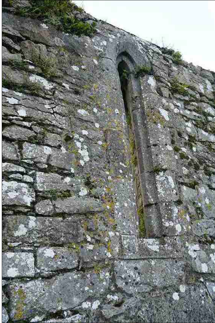
Figure 2.33. Window in N wall, from NE.
