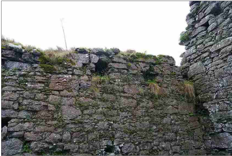
Figure 2.50. Joist holes in S wall, possible indication of a priest's residence, from N.
