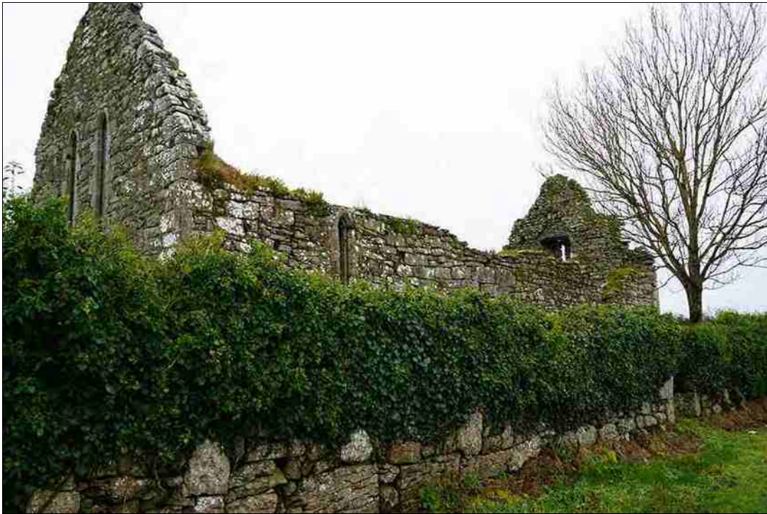
Figure 2.15. View of church from NE.
