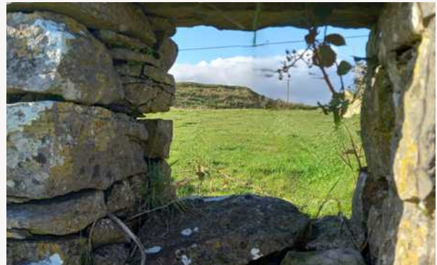
A view through a built-in sheep creep within a vernacular dry stone wall field boundary, towards the fine platform earthwork of Rathmore, Rathcroghan, Co. Roscommon.
