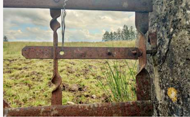
A traditional vernacular wrought iron gate lock with decorative twists, still in use, at Rathcroghan Co. Roscommon.
