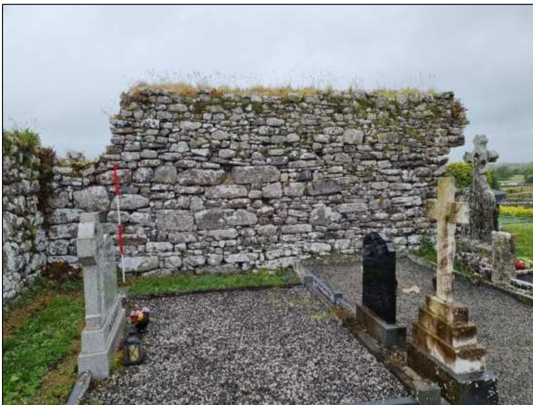
Plate 3: General view of the north wall looking north.
