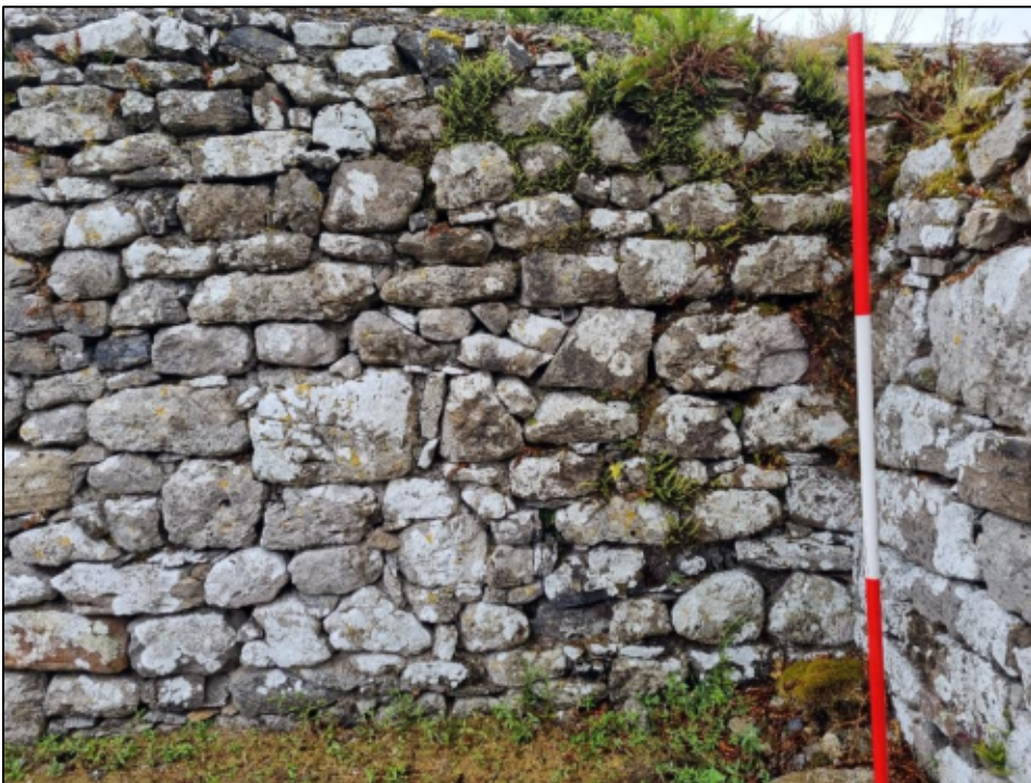
Plate 5: Junction of the wall enclosing the vault (fifteenth-century) with the north wall (eighteenth-century reconstruction).
