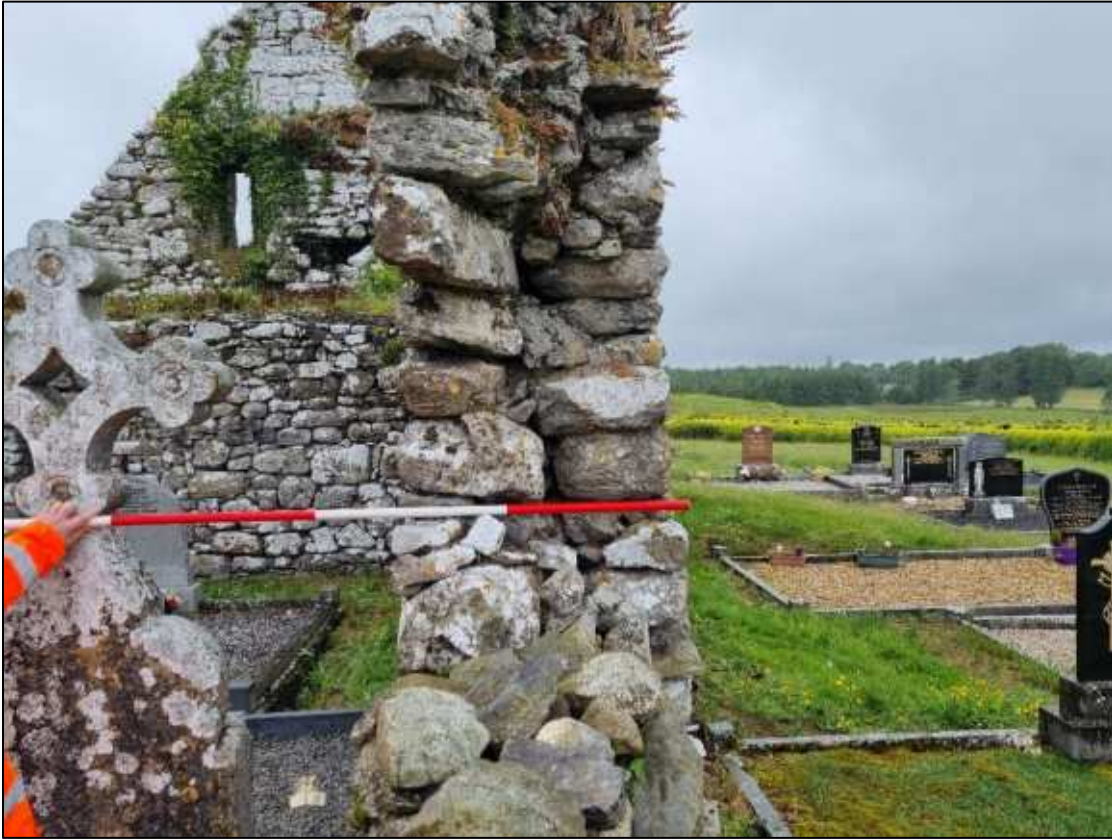
Plate 26: The wall is about 800mm thick.
