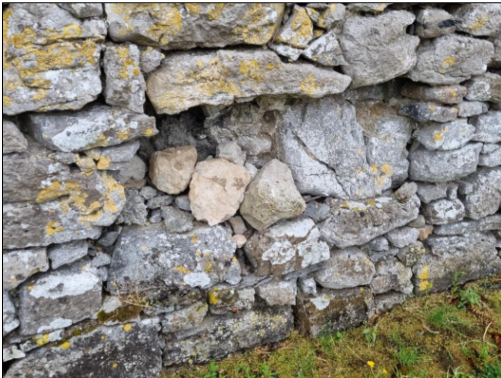
Plate 21: Some elements of the north wall looking south require minor rebuilding and pinning stones will be required in the pointing exercise.
