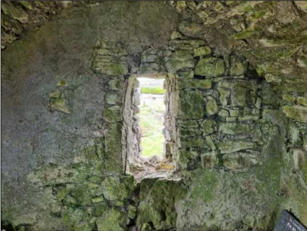
Plate 10: Window in south wall.
