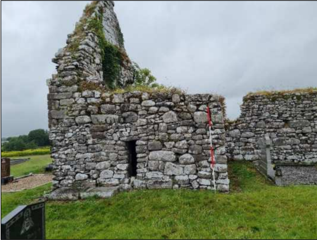
Plate 17: South elevation, overview of the building looking north.
