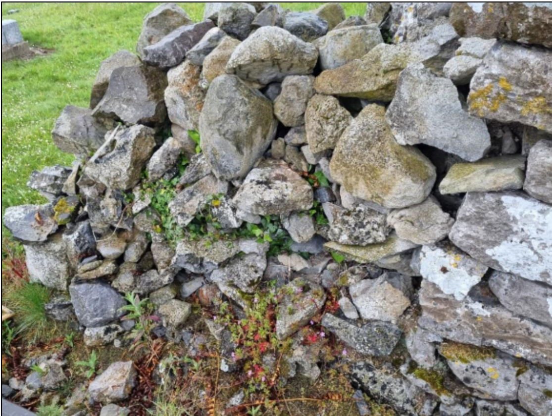
Plate 25: The end section of recent drystone walling is to remain.
