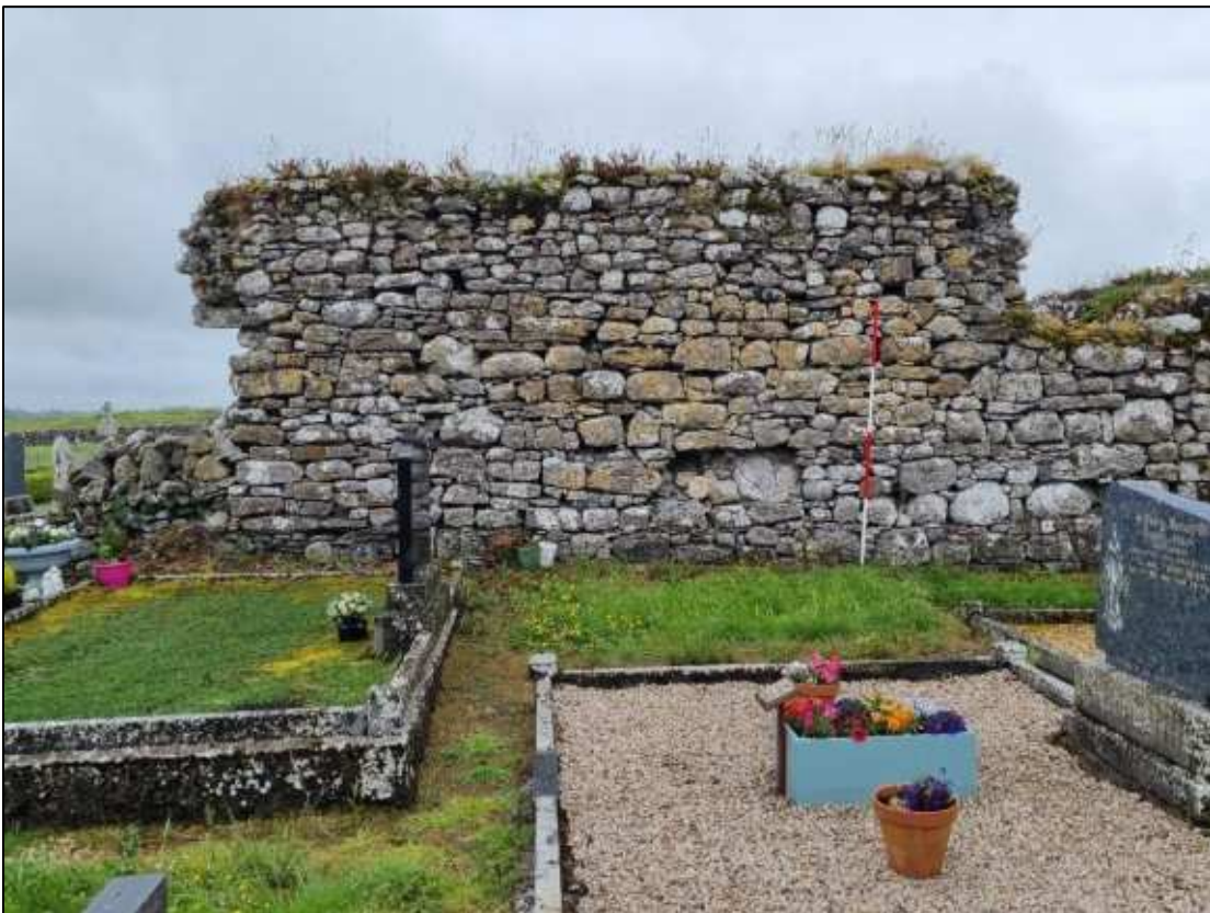
Plate 24: Overview of the north wall looking south.
