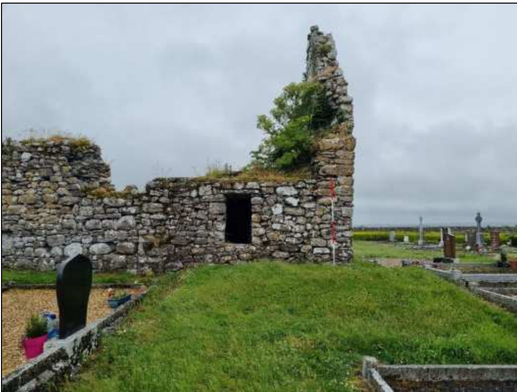
Plate 20: Overview of building looking south.
