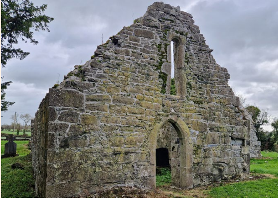
The western gable with off-centre window. (Photo credit: Bernie Doherty)
