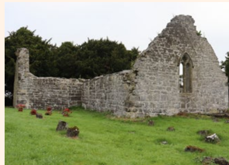
South gable after conservation works. (Photo credit: Bernie Doherty)
