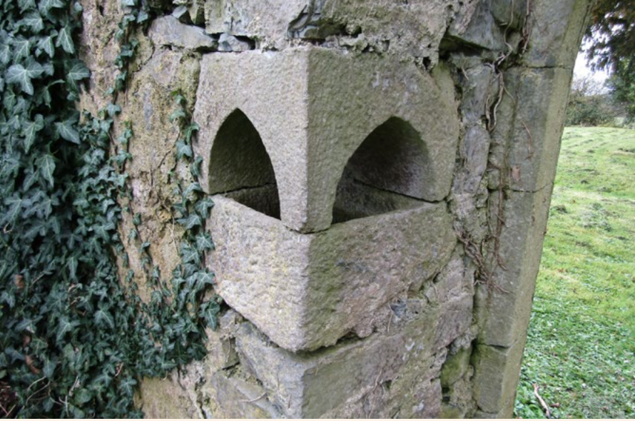
A medieval-designed font/stoup is built within the interior wall. (Photo credit: Dominic Delany)
