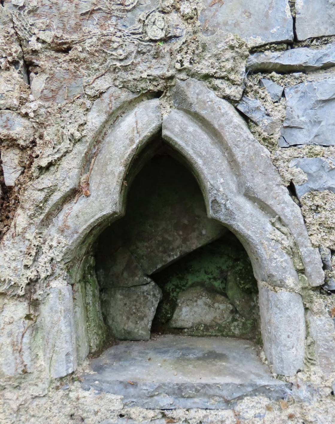
Piscina after conservation works. (Photo credit: Dominic Delany)
