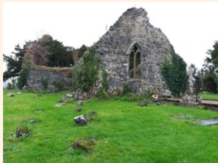
South gable before conservation works. (Photo credit: Bernie Doherty)
