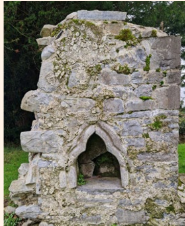
Piscina after conservation works. (Photo credit: Bernie Doherty)
