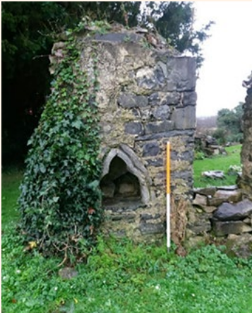
Piscina prior to conservation works. (Photo credit: Bernie Doherty)
