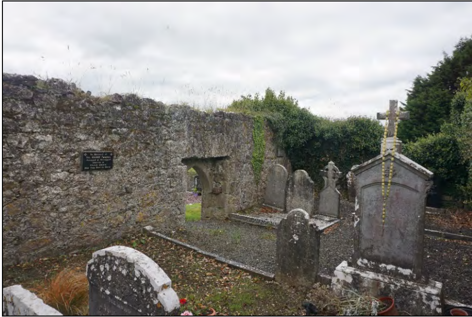
Photograph 12 Internal view of the southern elevation.
