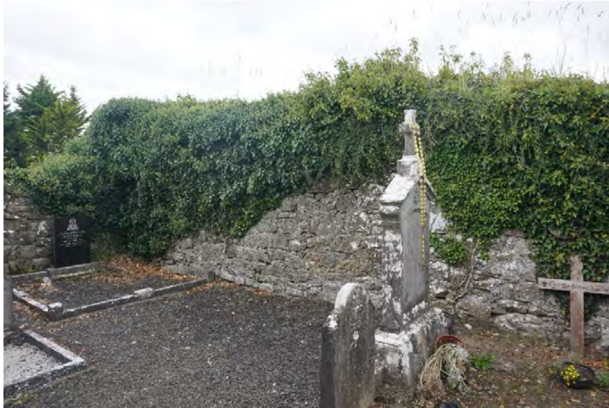
Photograph 4 Internal view of the northern wall, western end.
