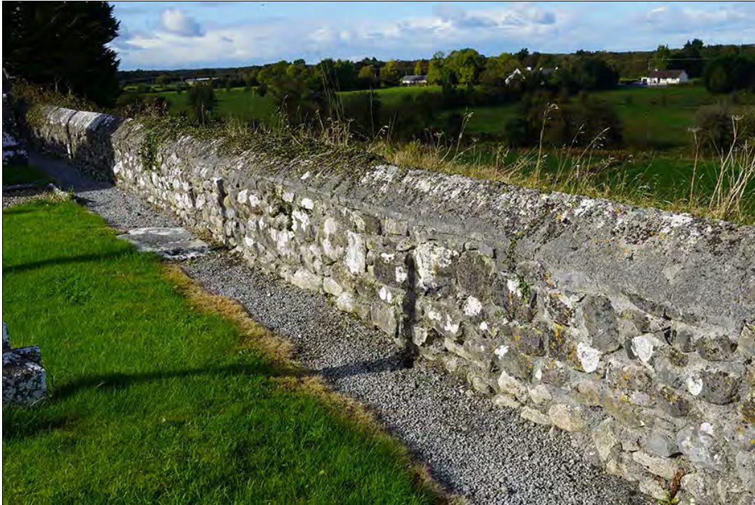
Figure 2.67. Graveyard wall at N, from E (F. Coyne).
