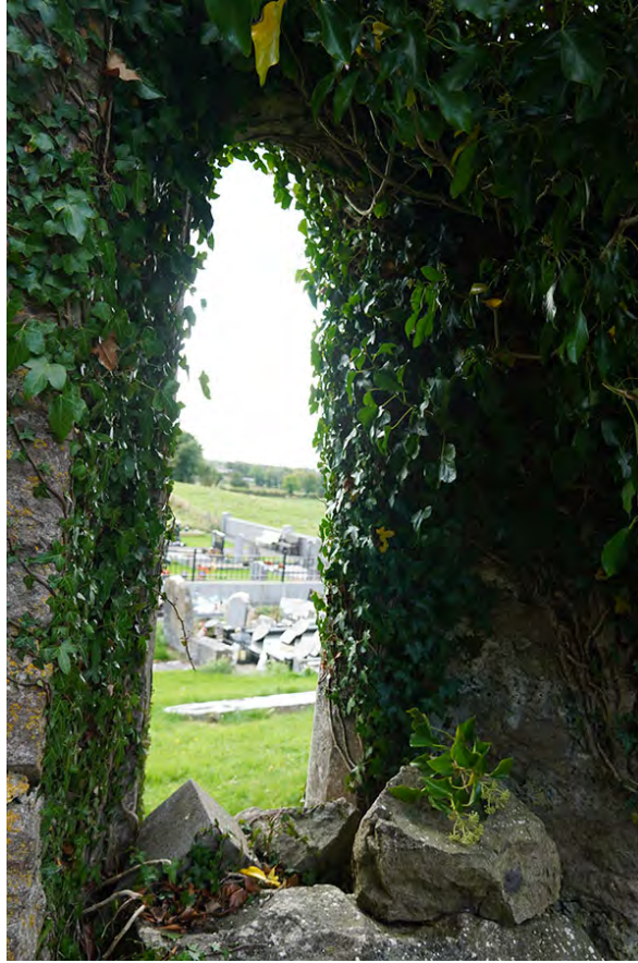
Figure 2.50. Internal view of south window, from N (F. Coyne).
