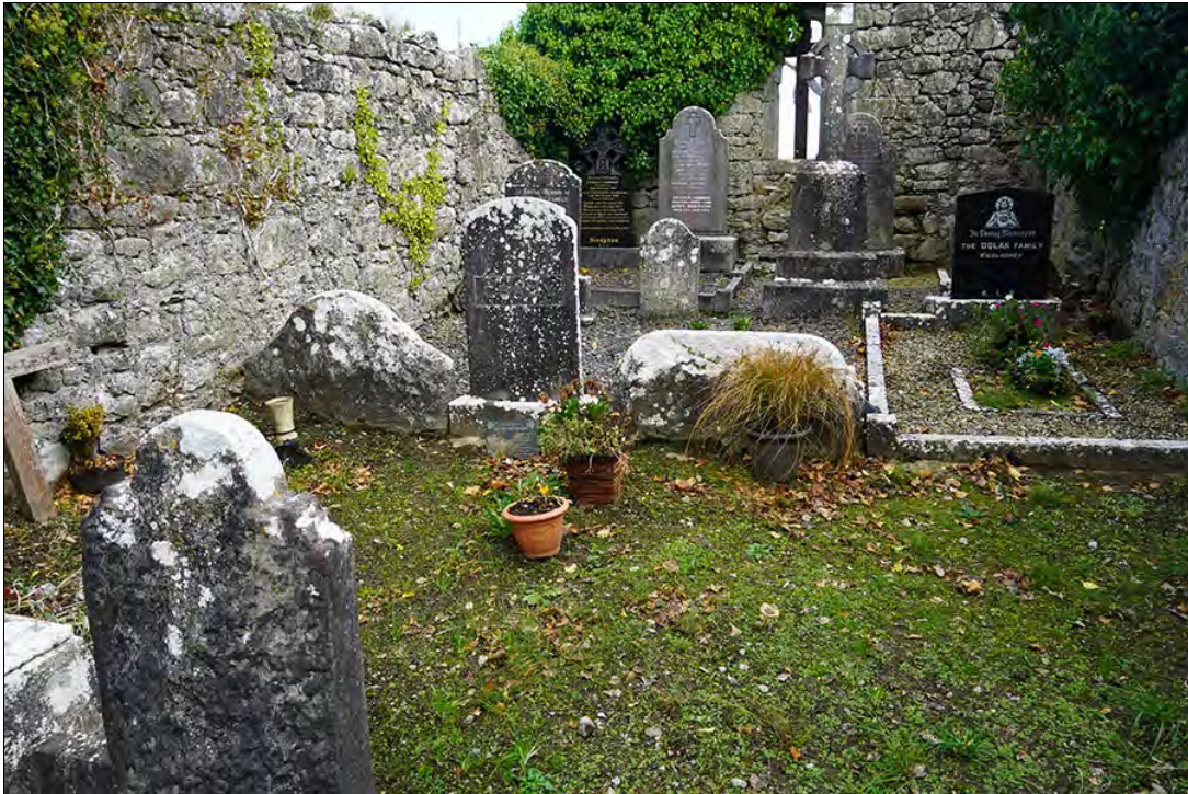
Figure 2.25. Graves in the interior of the E side of church, from W (F. Coyne).
