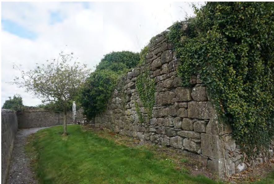
Photograph 5 View of the western wall.
