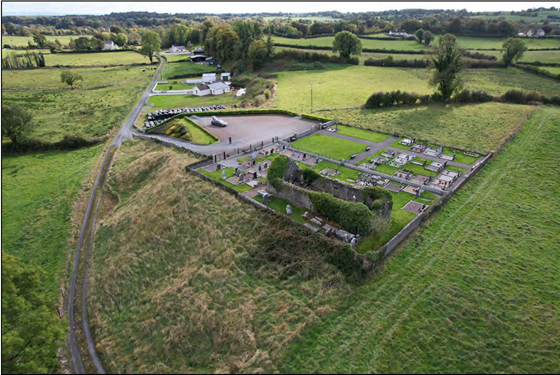
Figure 2.5. Aerial view of site looking northeast (F. Coyne).
