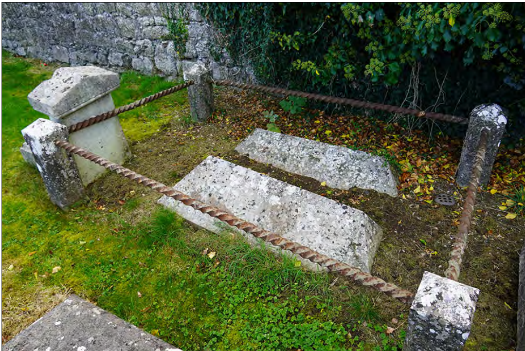
Figure 2.30. 20 th century cast iron and concrete surround for 18/19 hogs back graves, from NW (F. Coyne).
