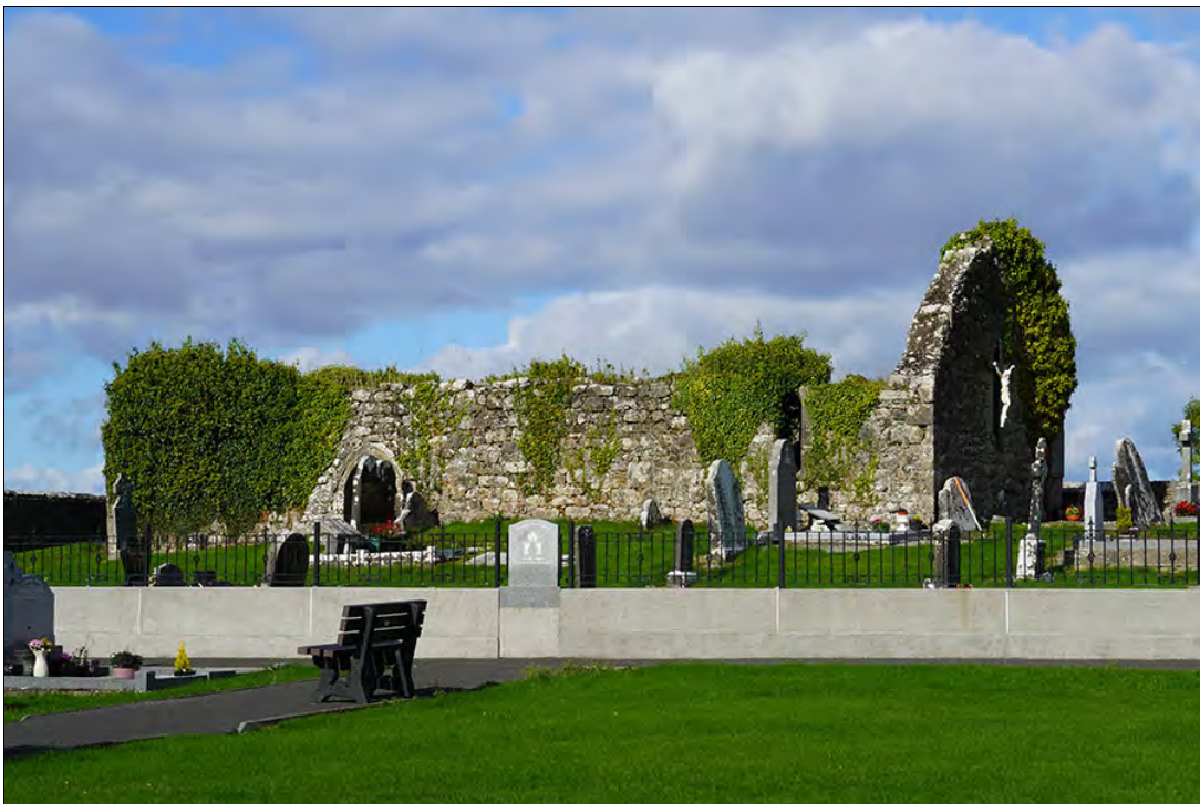
Figure 2.68. Modern block wall and railings graveyard wall, from S (F. Coyne).
