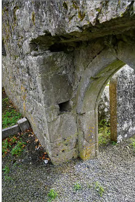
Figure 2.58. Drawbar socket on internal side of door, from NW (F. Coyne).
