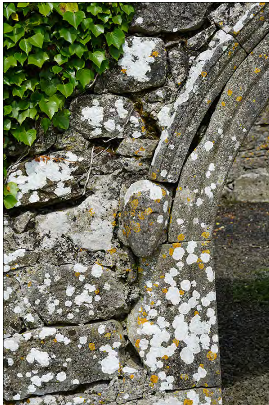
Figure 2.53. Stone head label stop on W side of door, from S (F. Coyne).
