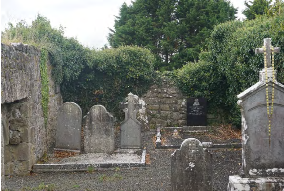
Photograph 6 Internal view of the western wall. Mostly covered in ivy.
