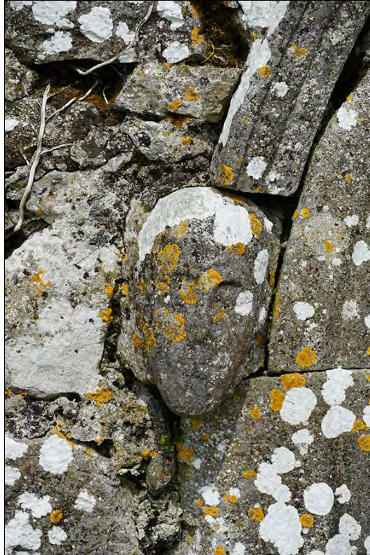
Figure 2.54. Detail of stone head label stop on W side of door, from S (F. Coyne).
