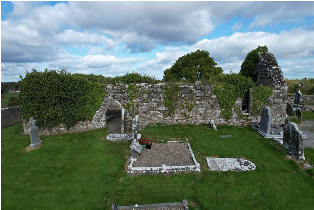
Figure 2.49. S wall of church, from S (F. Coyne).
