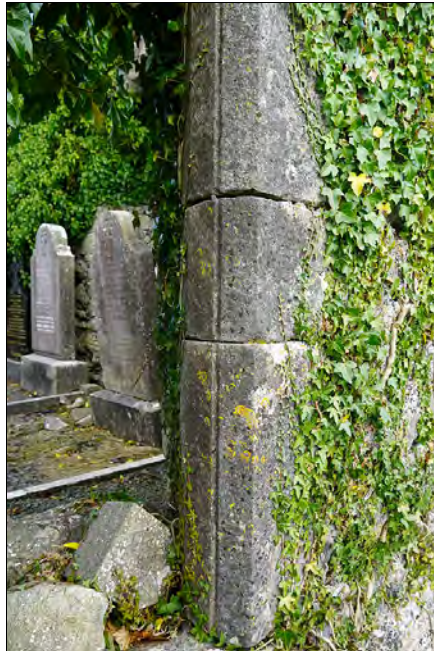
Figure 2.51. External view of rebate for glazing on south window, from S (F. Coyne).
