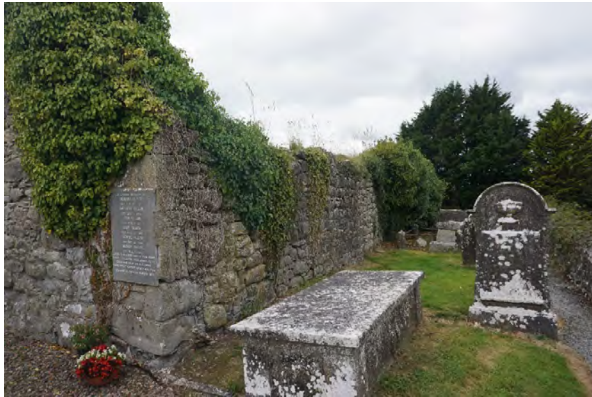
Figure View of the northern elevation of St. Grellan's Church.
