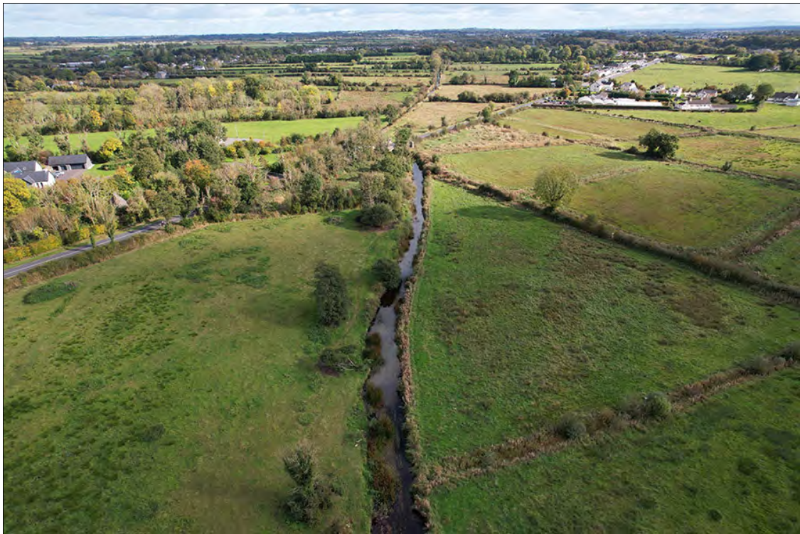
Figure 2.6. Aerial view of Deerpark River, from W (F. Coyne).
