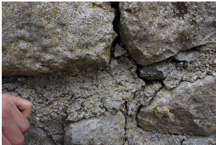
Photograph 14 Detail of remedial cementitious binder.
