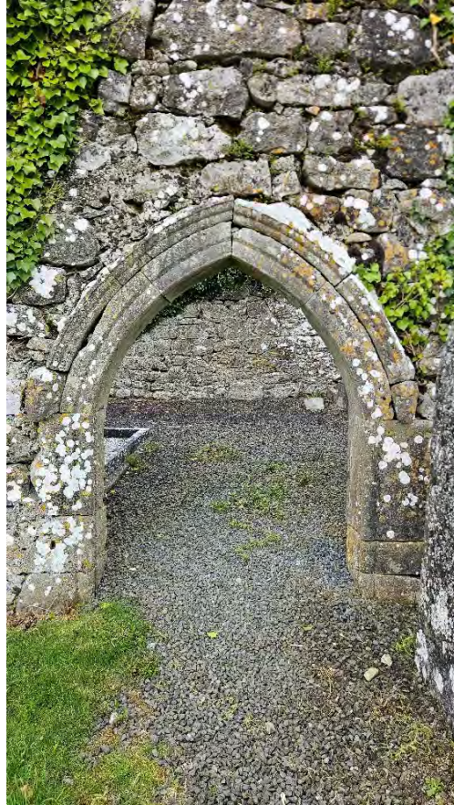
Photograph 10 Lancet arched door opening. The masonry units are in good repair.
