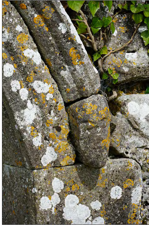
Figure 2.56. Detail of stone head label stop on E side of door, from S (F. Coyne).
