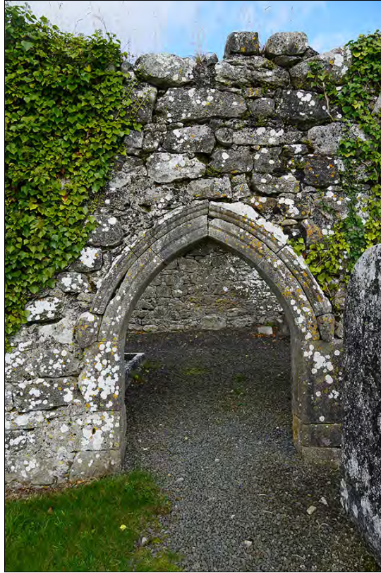
Figure 2.52. External view of door in S wall, from S (F. Coyne).
