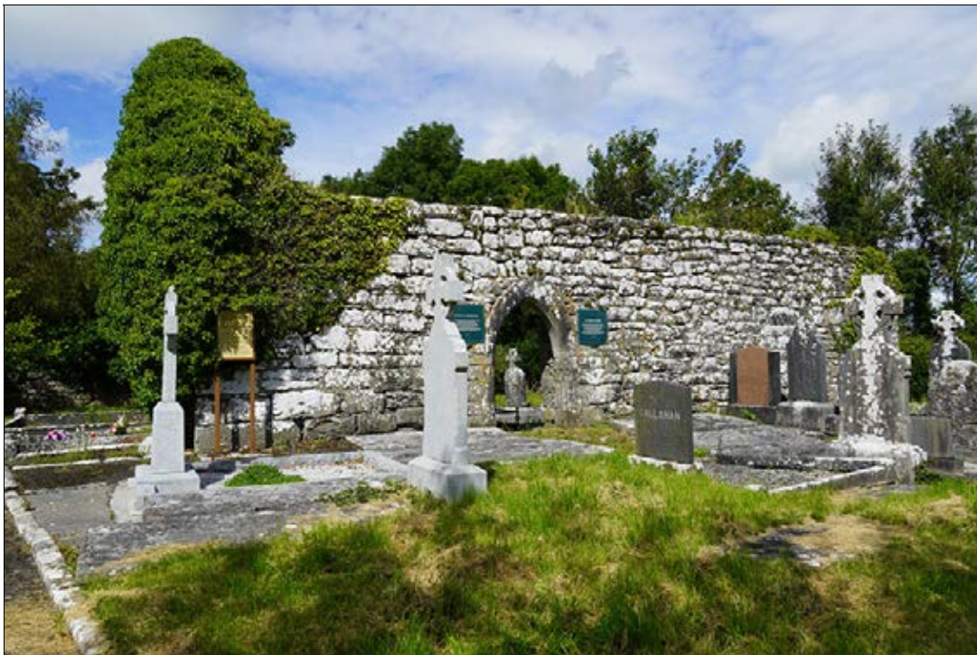
Figure 2.29. South wall and west gable, from SW.
