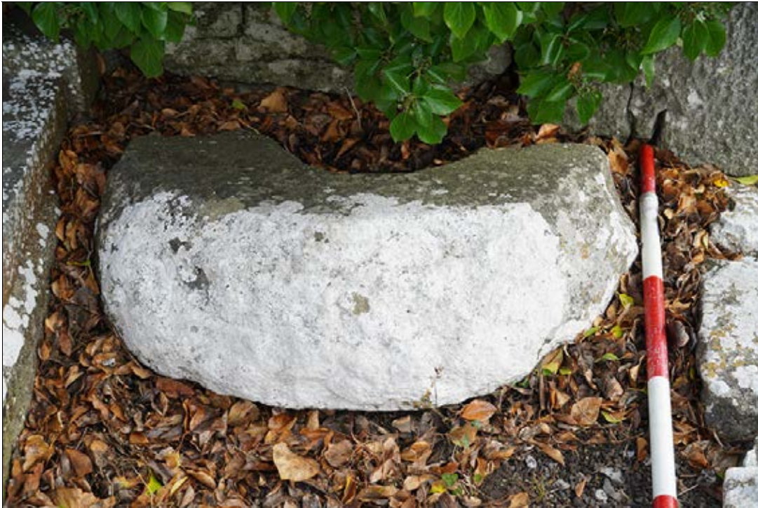
Figure 2.35. 12 th /13 th century window head fragment at W gable of church, from W
