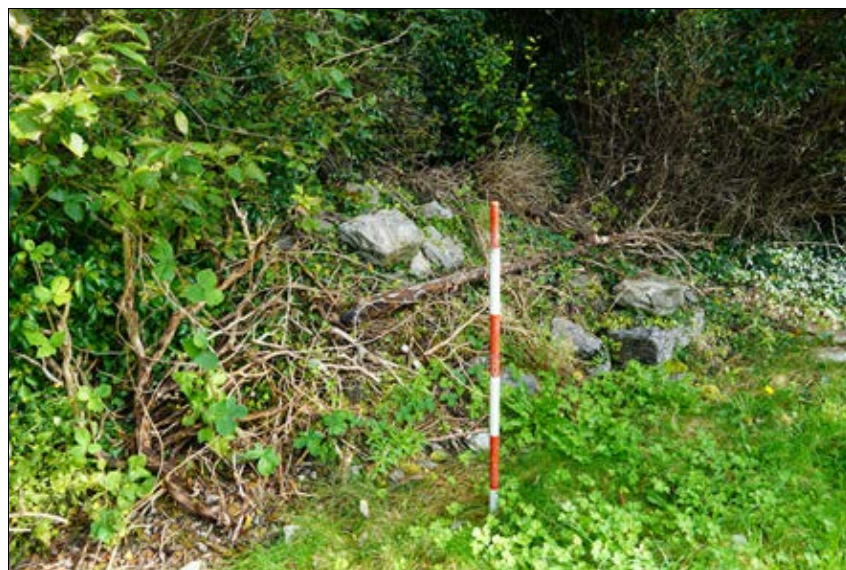
Figure 2.40. Stone pile, collapsed wall of graveyard at N, from SW.
