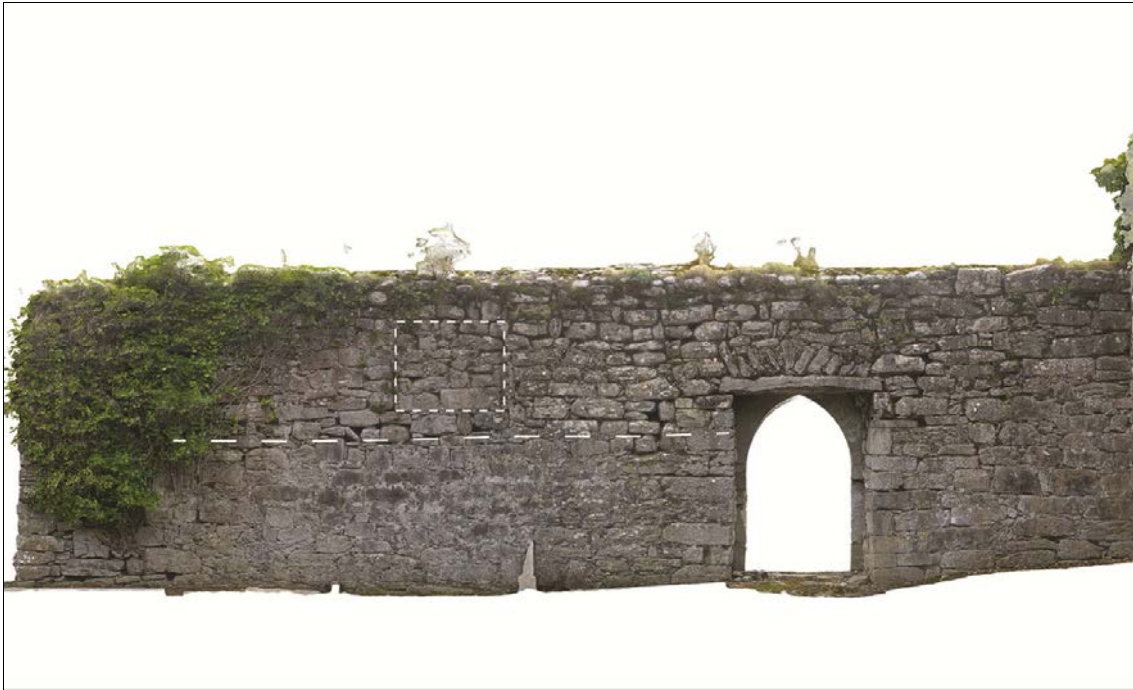
Figure 2.14. Elevation of interior of church wall (after KGSS, annotated by writer)
