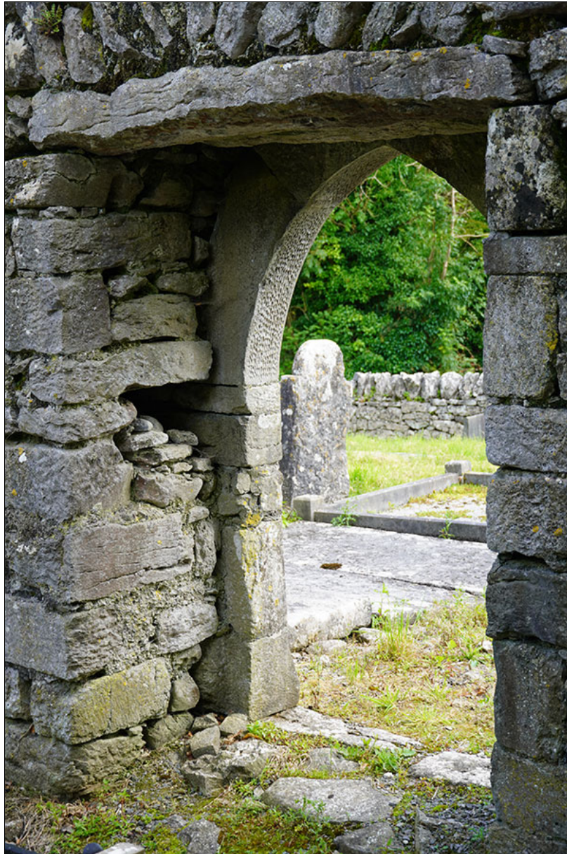
Figure 2.32. Church door, note drawbar hole, and 15 th century pointed archway with punch dressing, from interior of church, from NW
