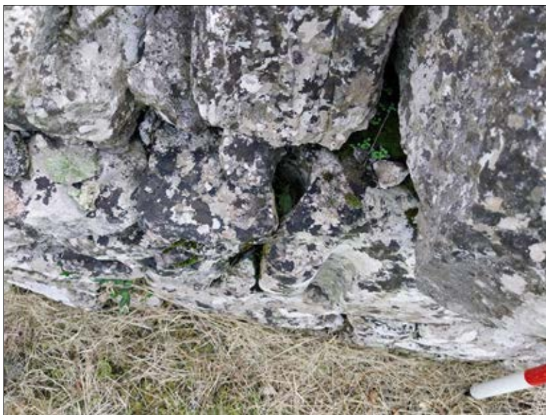
Figure 2.37. 12 th /13 th century window fragment in wall, from N.
