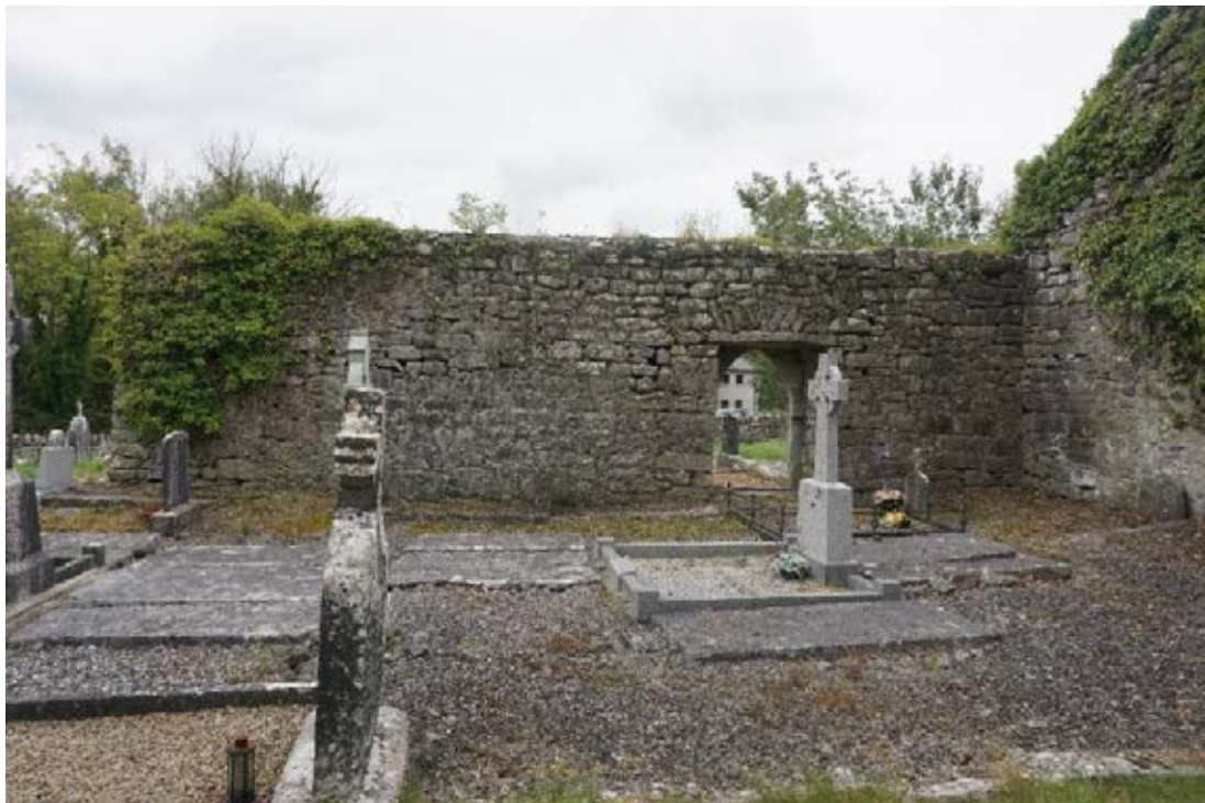
Photograph 5 Southern Wall internal façade.
