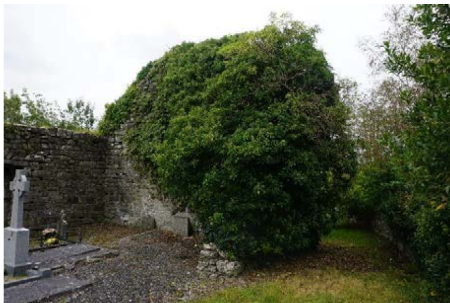
Photograph 2 Interior façade of the western gable.
