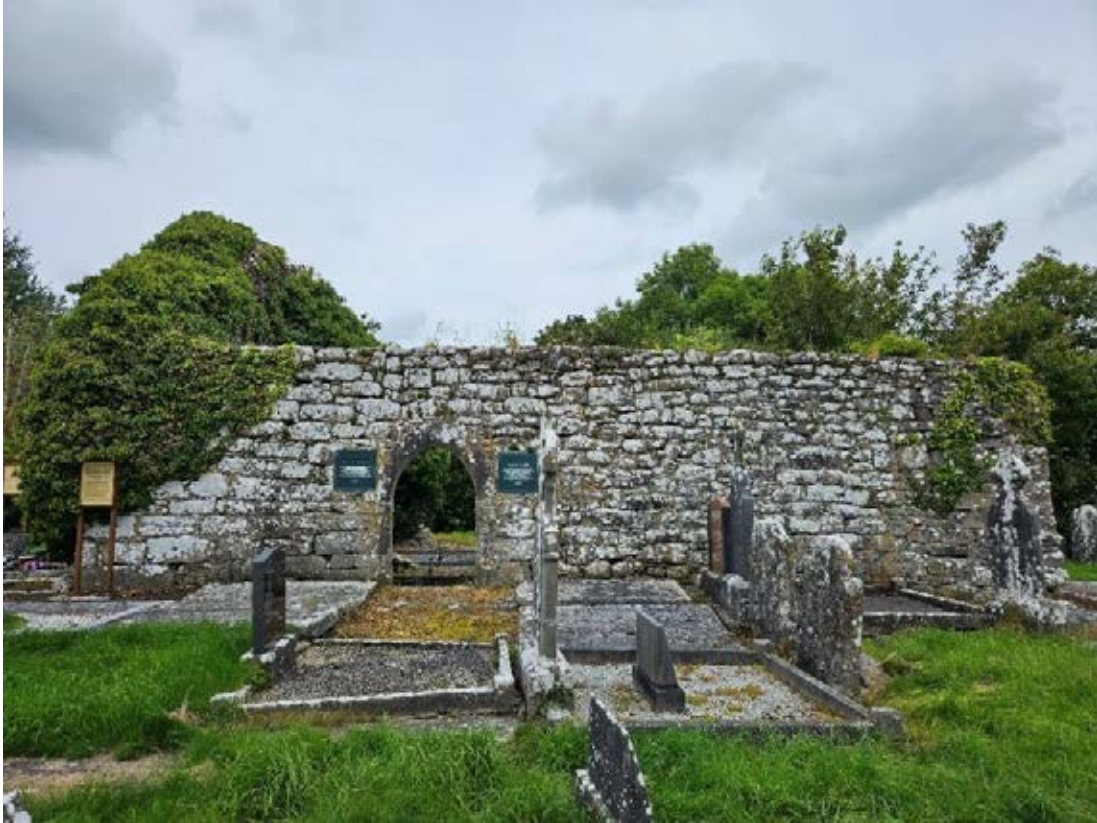
Photograph 4 Southern wall external façade.
