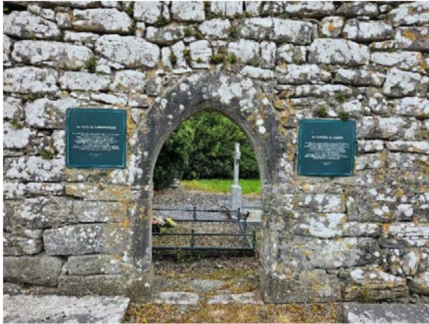
Photograph 6 Detail of the surviving door opening.
