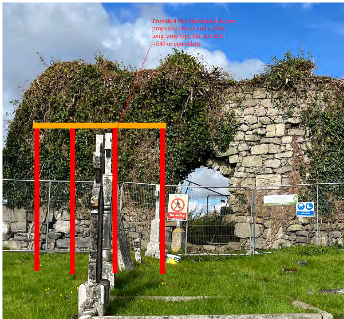
Figure 4 Location of propping
