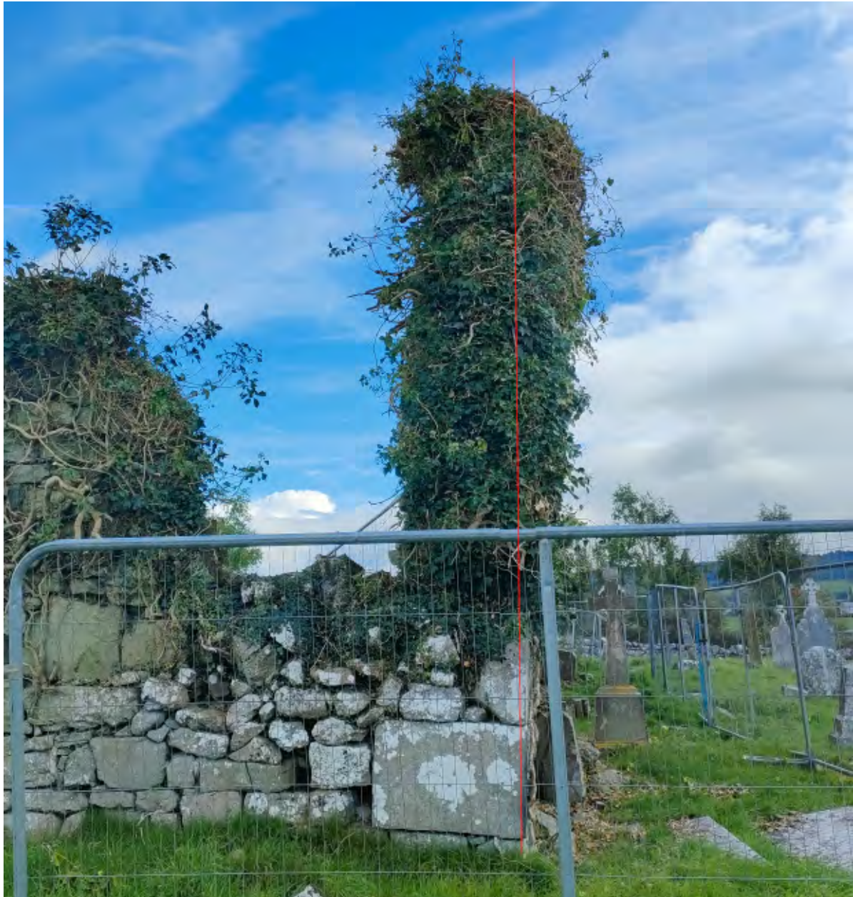
Figure 1 Lean on the wall is evident
