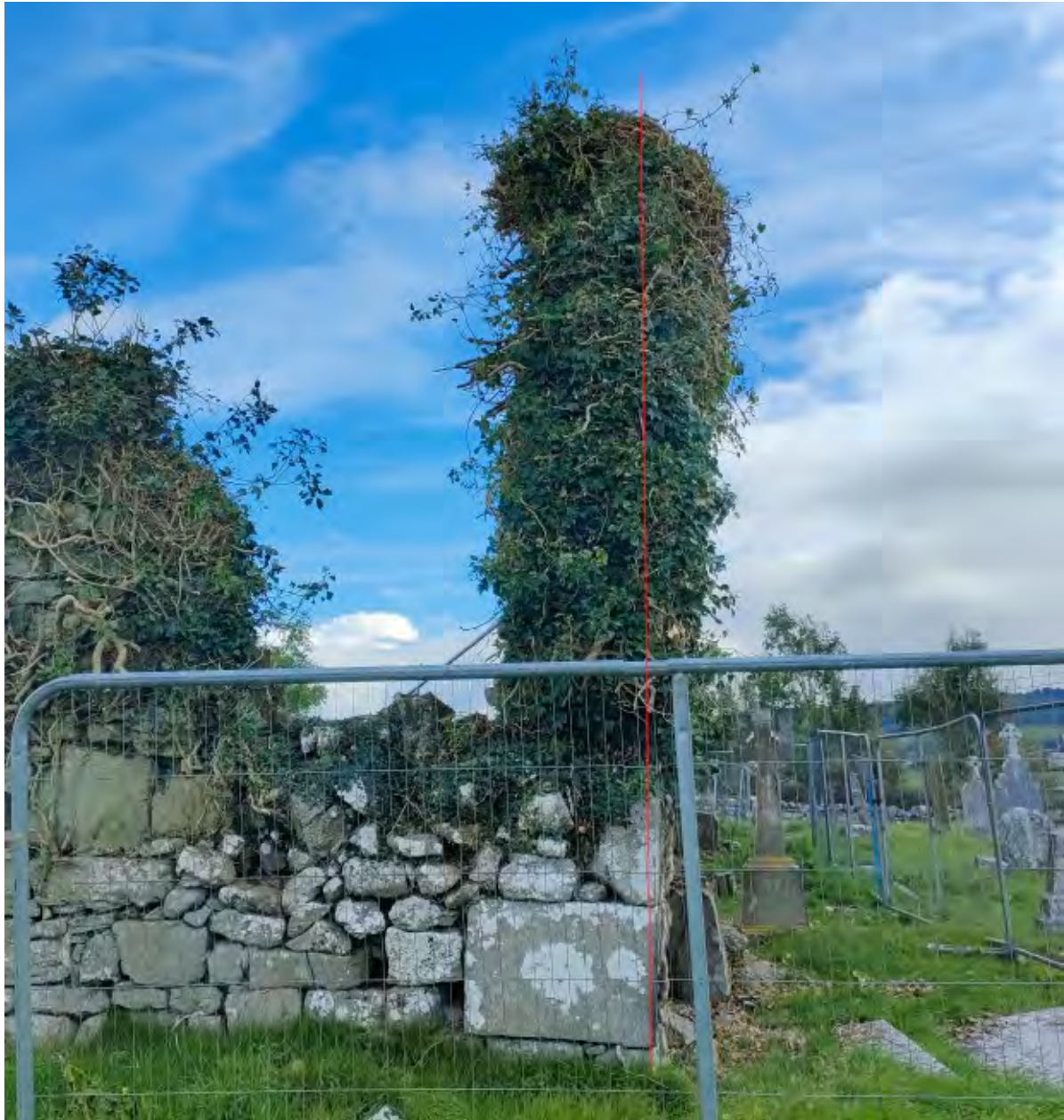
Figure 1 Lean on the wall is evident
