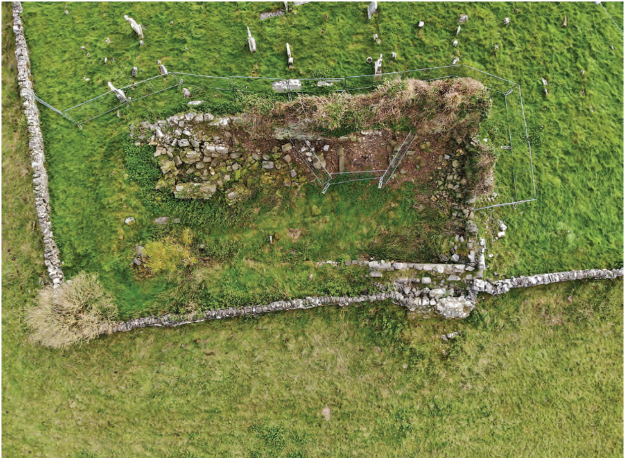
Figure 3 - Aerial view of the church, a single cell structure - the east wall (on left of photo) is entirely collapsed
