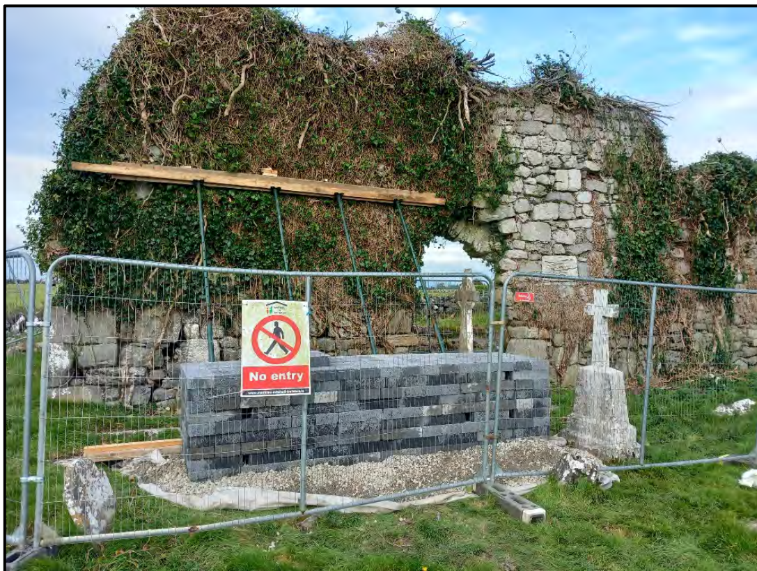
Plate 19: Looking North showing south wall propped as per specifications from John Britton, Structural Engineer, approved by NMS, Department of Housing, Local Government & Heritage
