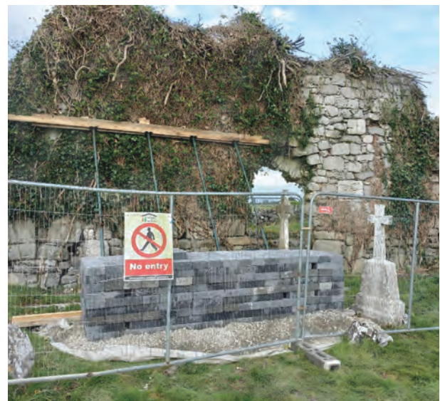
Figure 20 - Installation of propping underway at Issertkelly
