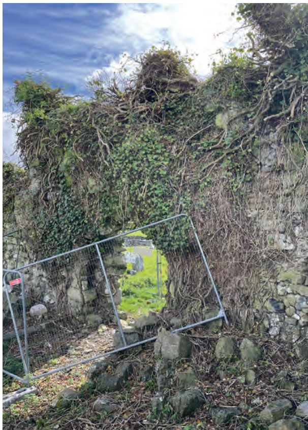
Figure 24 - Large vegetation still rooted into the top of the wall
