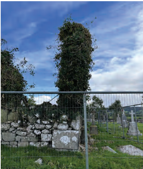
Figure 15 - Lean of the south wall is evident when viewed from the side
