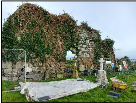
Plate 17 Looking north east showing terram on surface to protect ground beneath stone base. Plate 18 Stone on terram.
