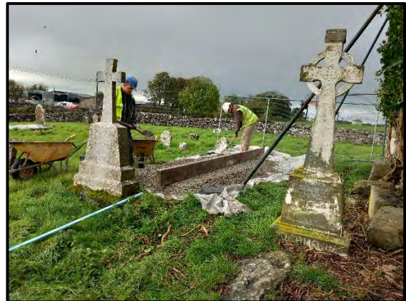
Plate 17 Looking north east showing terram on surface to protect ground beneath stone base. Plate 18 Stone on terram.
