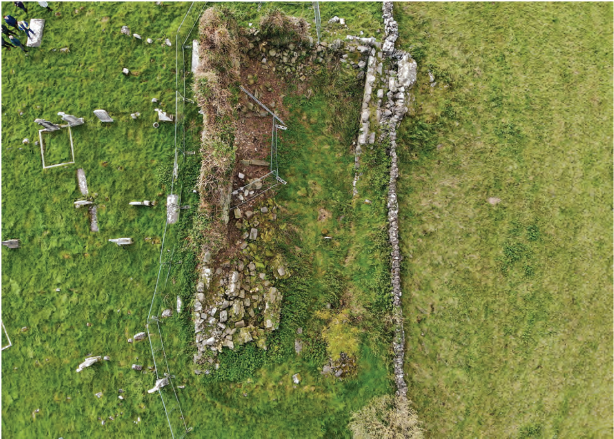
Figure 12 - The north wall (on right in photo) has collapsed in part onto the boundary wall
