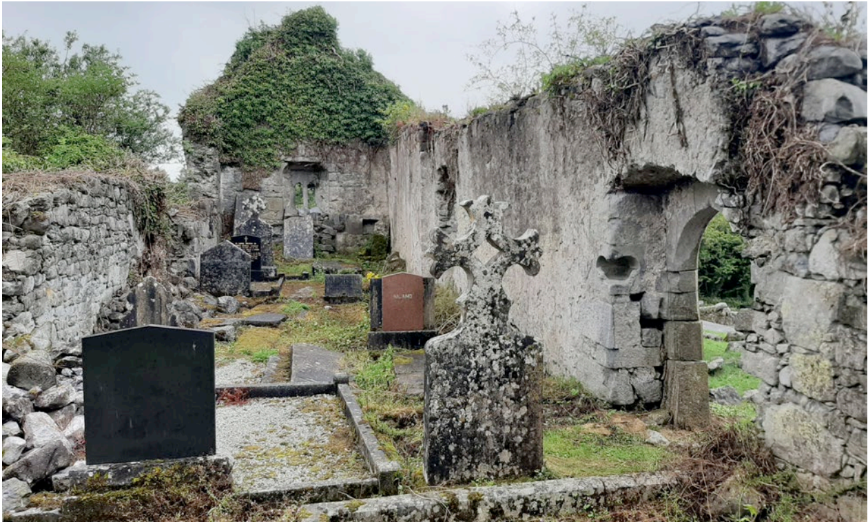
General view of church interior, looking East
