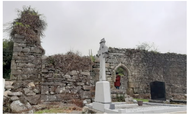
Viewing looking towards South wall, with West gable on the left
