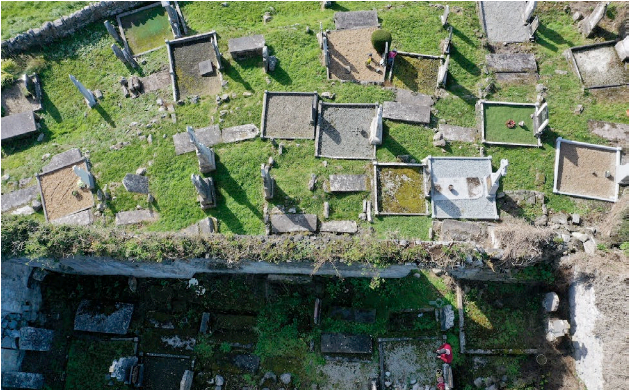
Aerial view looking directly down onto the South wall and graveyard south of the church
