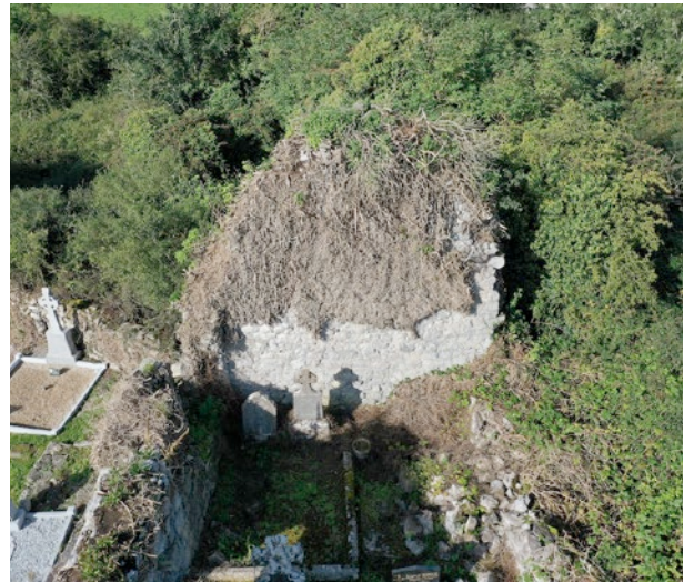
Aerial view looking onto West gable
