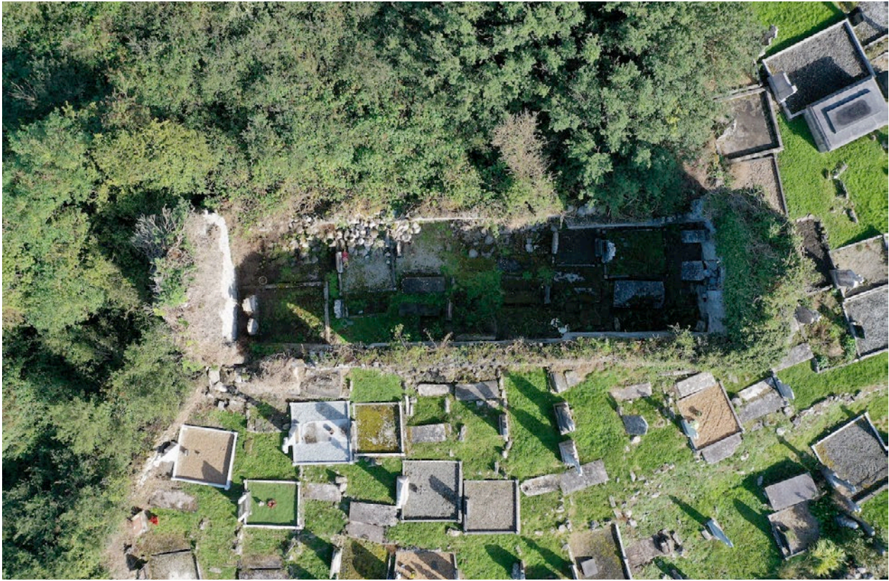
Aerial view looking directly down on the church, orientated North
