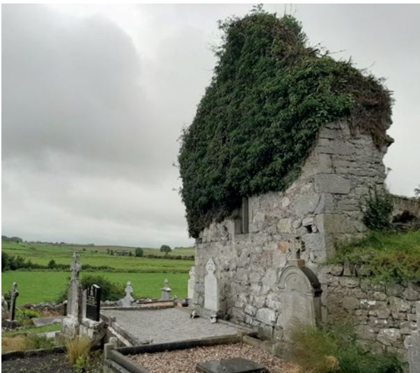
View looking South-West showing corner build up at East facade
