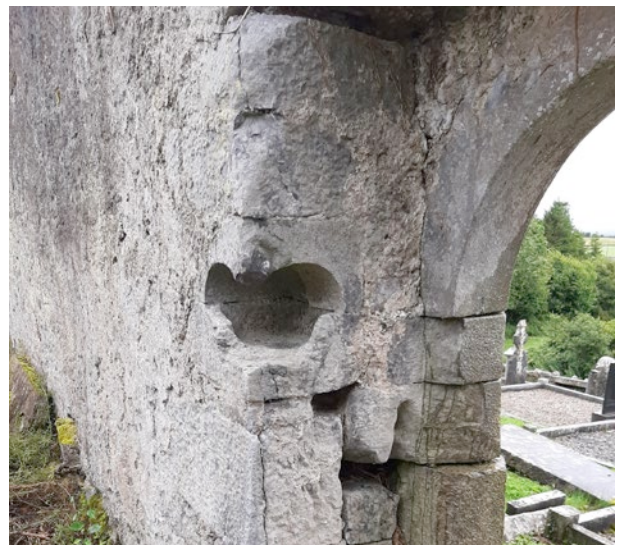
Internal view of water font detail within the entrance opening
