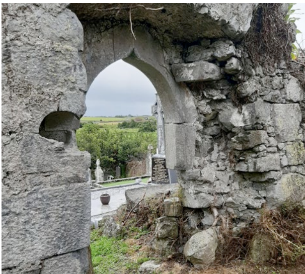
Internal view of entrance doorway
