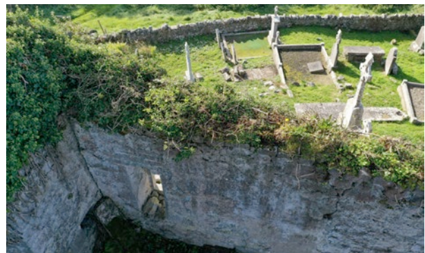
Aerial view of top of South wall
