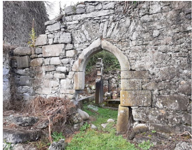
General view of the entrance to the church on South Elevation
