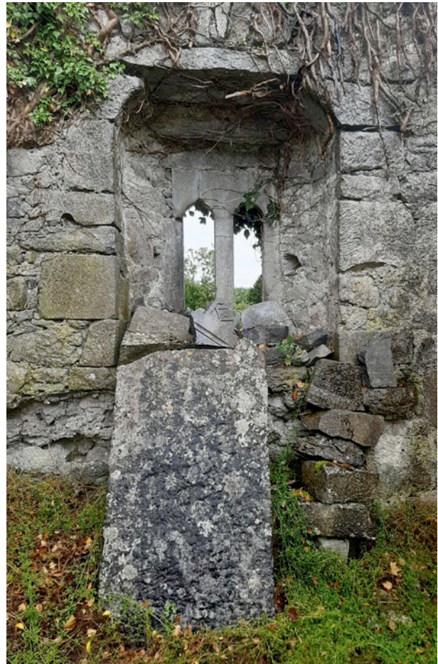
Internal view of East gable window
