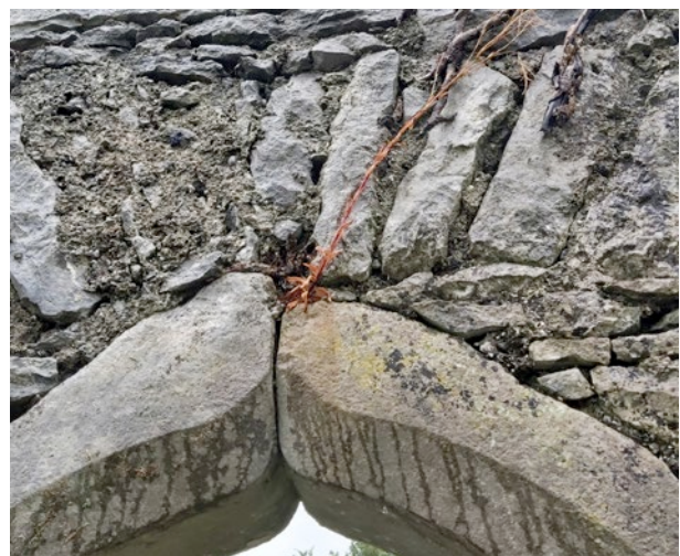
External view of stone detail above entrance door
