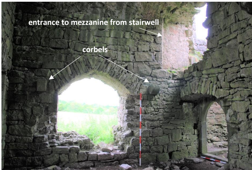
Fig. 24 Mezzanine beneath the vault reached from stairwell in southeast corner. Corbels for mezzanine floor beams can be seen in the east wall.
