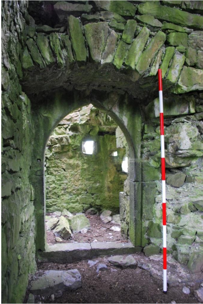
Fig. 21 Cut-stone, semi-pointed doorway leading from the stairwell space into the ground floor room.
