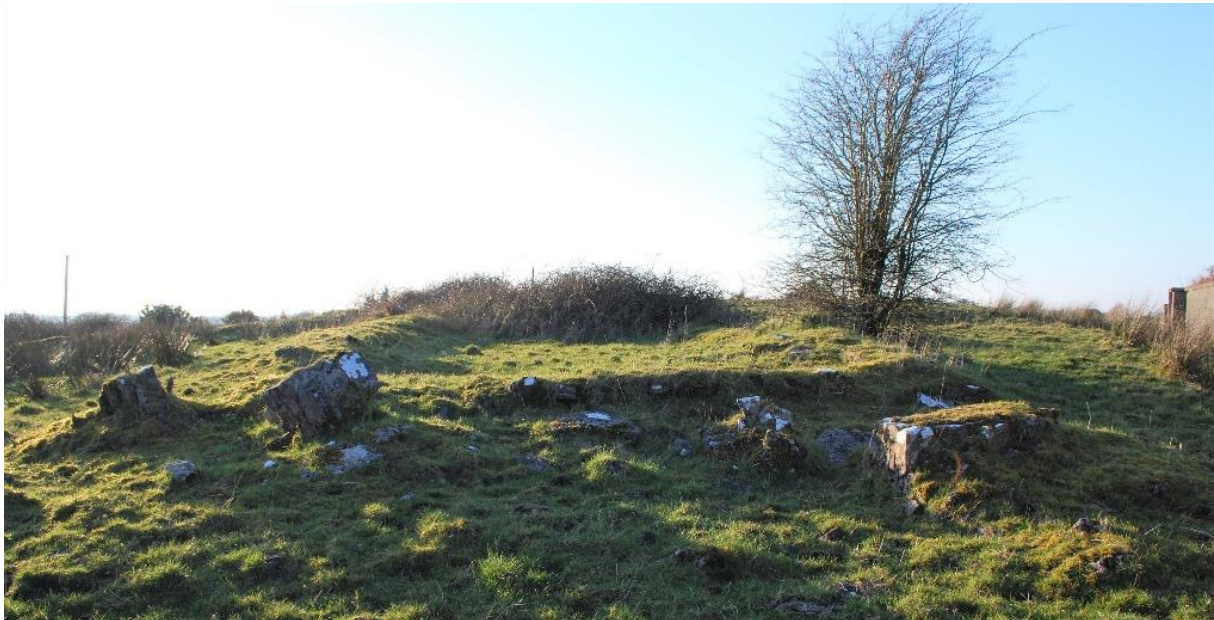
Fig. 35 Wall-footings of the building known as 'Kilcloony Church' viewed from east end.
