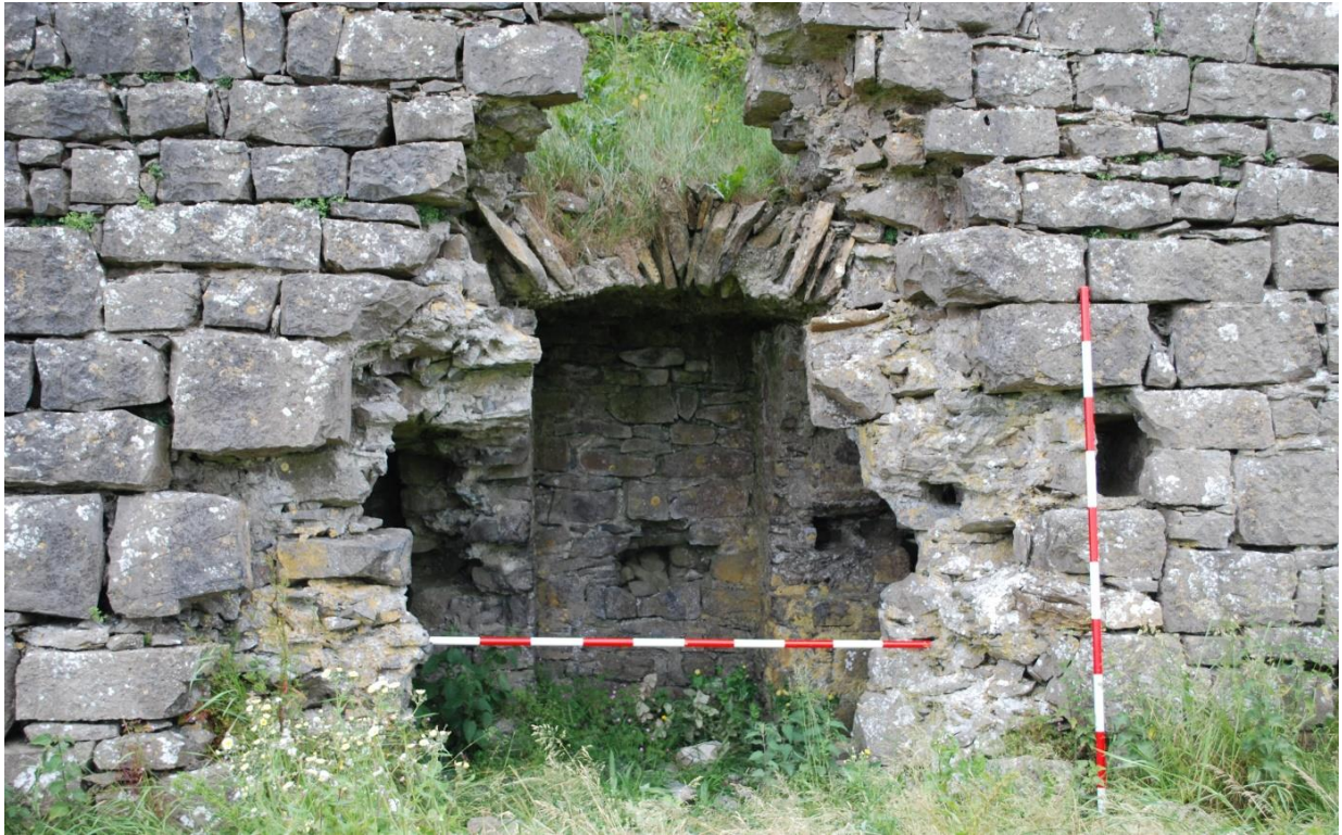
Fig. 13. The breached entrance in the south wall showing the lobby with its vaulted roof.
