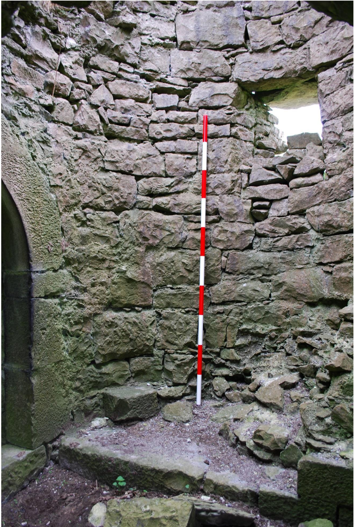
Fig. 19. Stairwell in southeast corner of the tower house.
