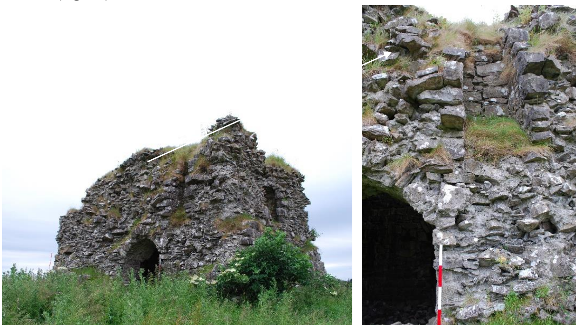
Fig. 30 The exposed garderobe chute at the north end of the east wall.
