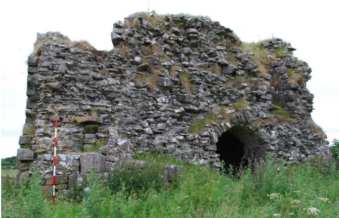
Fig. 8. East wall showing robbed-out masonry, window embrasure and garderobe chute.
