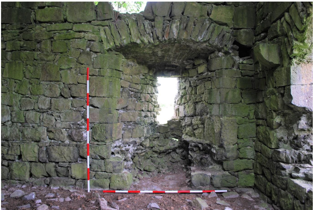
Fig. 23 Ground floor north wall with remains of single-light window and embrasure.
