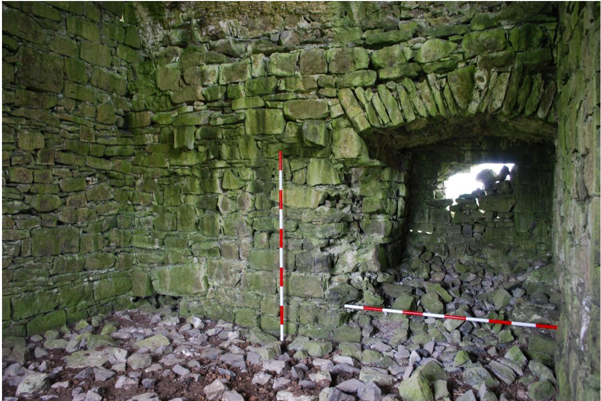
Fig. 22 Ground floor west wall with window embrasure.
