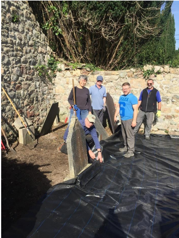
Laying membrane at church interior after week clearance.
