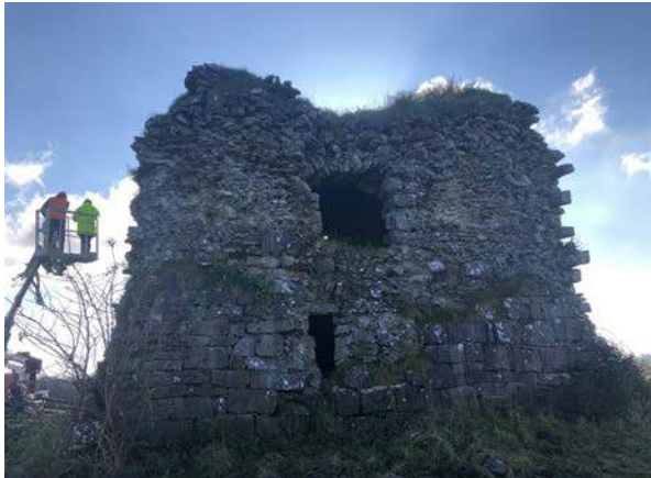
13. View of north west face.
