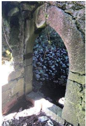
32. View of internal doorway.
