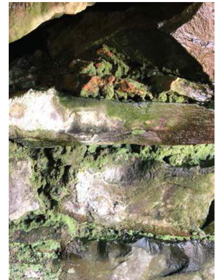
50. Detail of biofilm to alcove.
