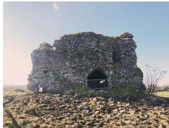
14. View of north east face showing temporary barricade.
