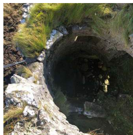
40. View down stairs showing thinness of wall in this location.
