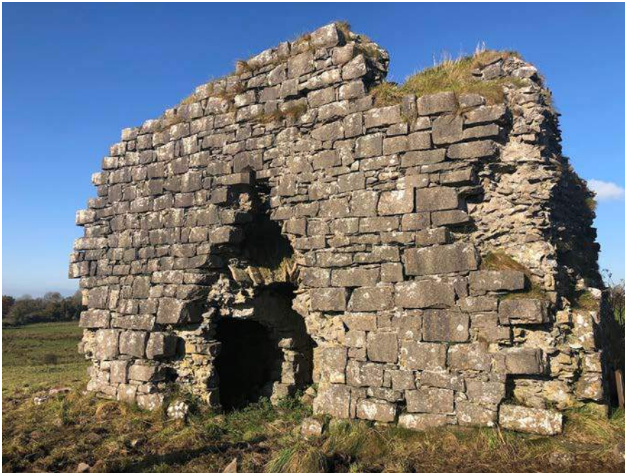
12. View of southeast face of tower and main entrance door.
