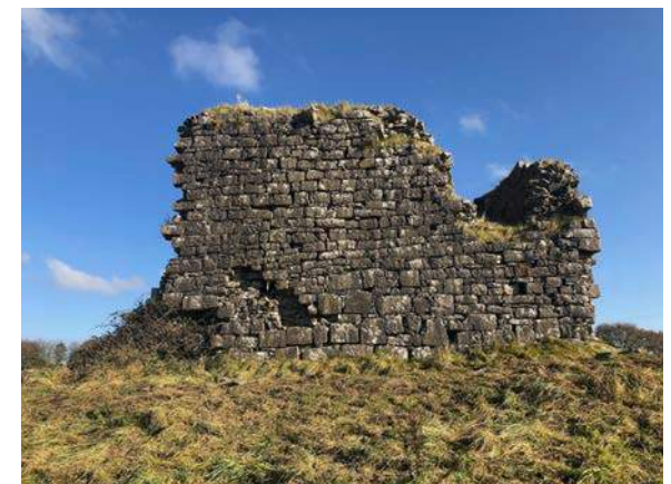
15. View of south west face.
