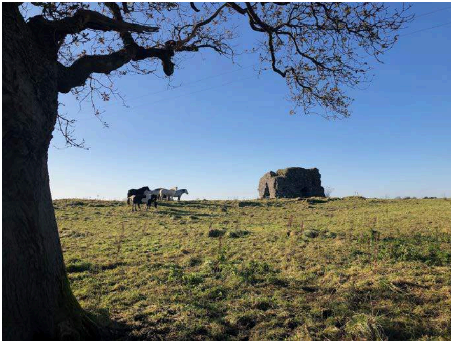
7. View of tower from approach to east.
