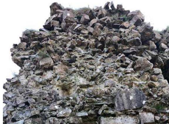
22. Detail of exposed wall core to north west face.
