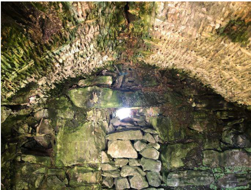
28. View of wickerwork centering to vault to chamber on ground level.
