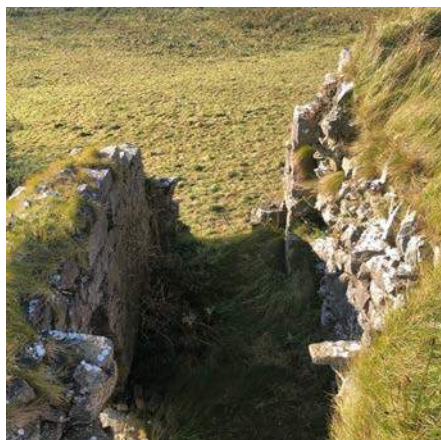
39. View overlooking subsidiary chamber showing badly eroded walls
