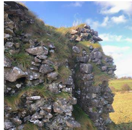
41. View of exposed garderobe chute to north east side.
