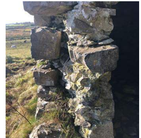
27. Detail showing cavity between facing stone to narrow front wall.
