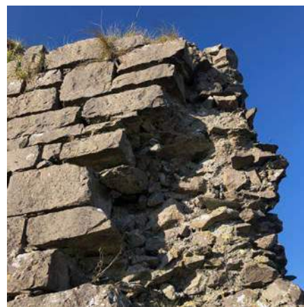
25. Detail of exposed wall core.
