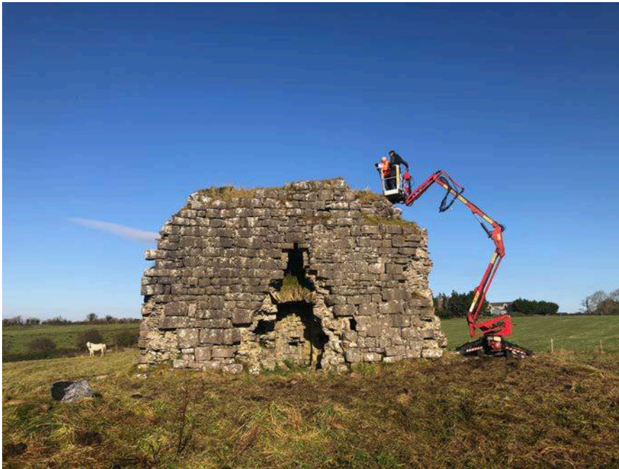
59. High level inspection of tower house underway in November 2020..
