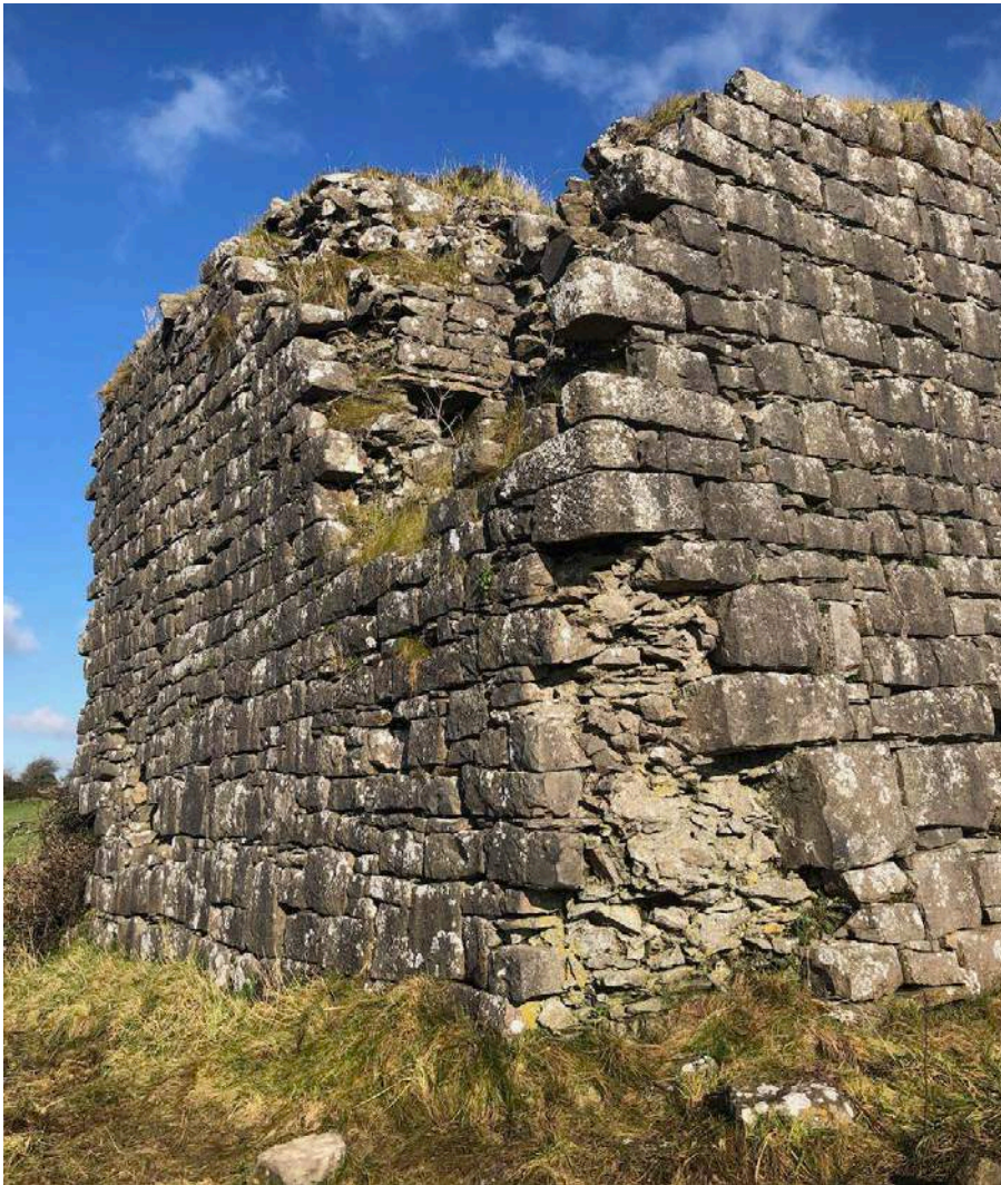
20. View of robbed-out corner to south of tower showing cantilevering quoins.
