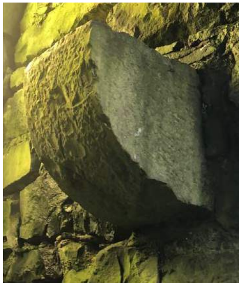
30. Detail of mezzanine corbel.
