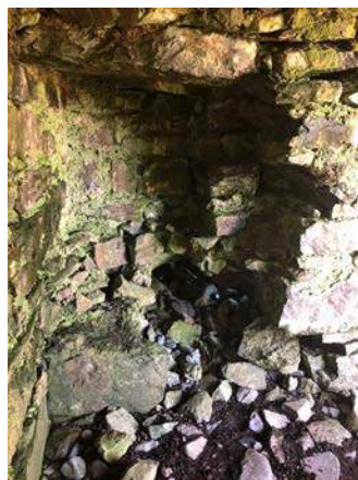
33. View of alcove with void to base of wall.
