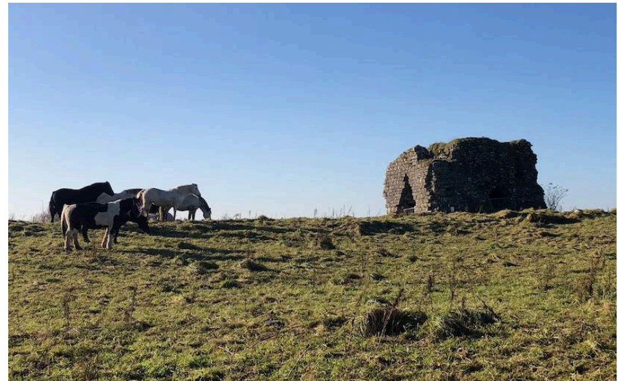
51. View of tower house and livestock from east.
